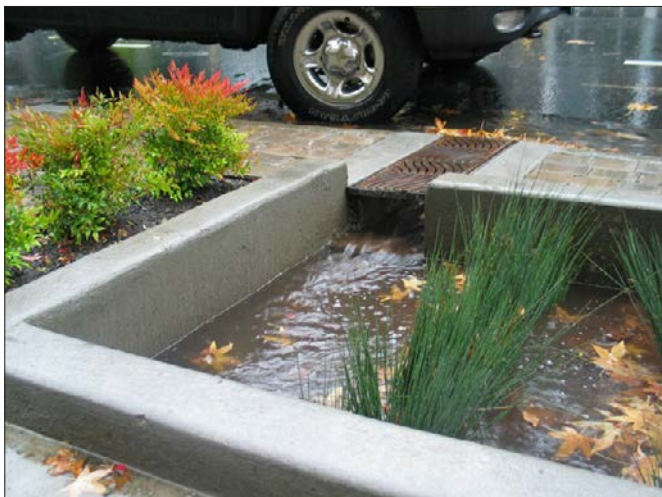
Figure 8 - A retrofitted ground-level raingarden, reducing water runoff into nearby waterways and filtering pollutants from stormwater
