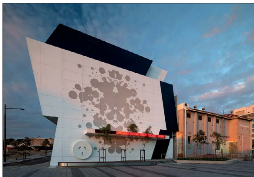
Figure 3 - Dandenong's 'Energy Centre' containing tri-generation facilities
