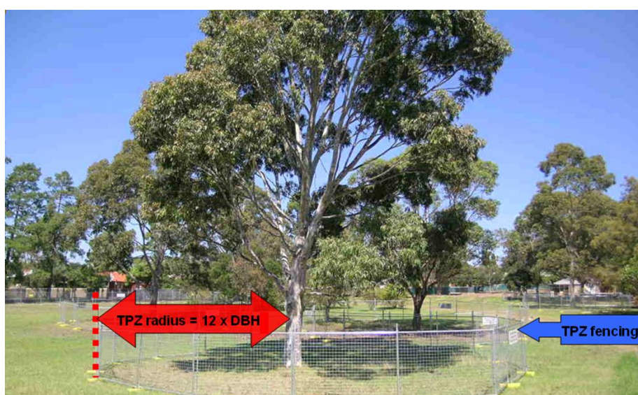
Figure 3: TPZ fencing is erected around retained trees prior to site works.
