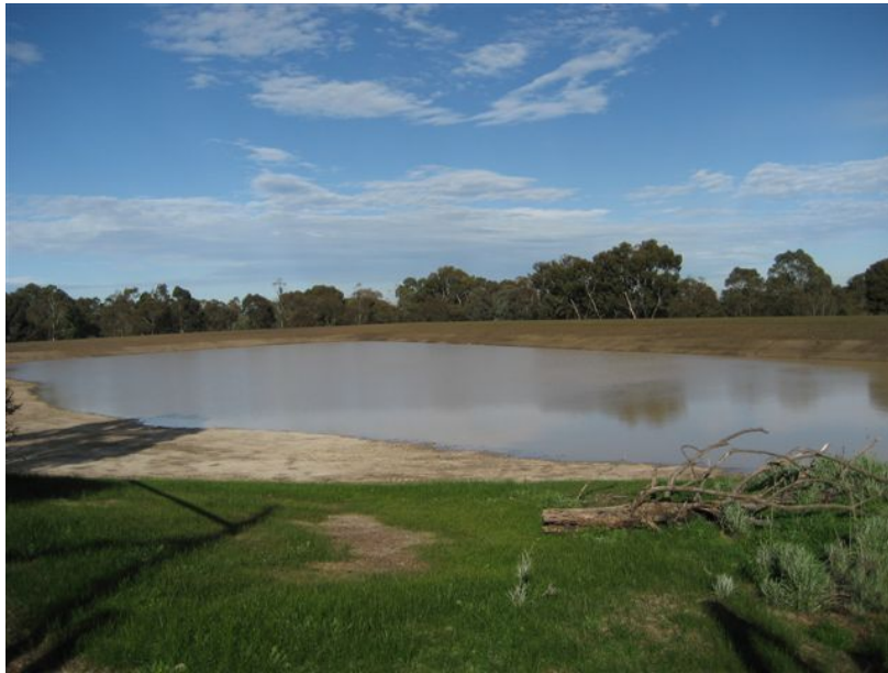
The newly constructed dam at Bundoora Park
