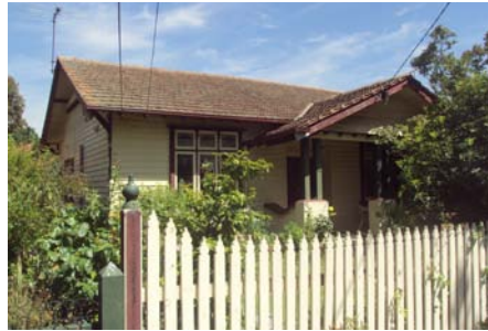
Figure 7 (left) A 1920s timber bungalow at 29 Naroon Road.
