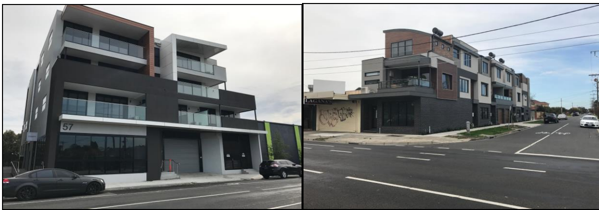
Figure 2: 57 and 23 Johnson Street
