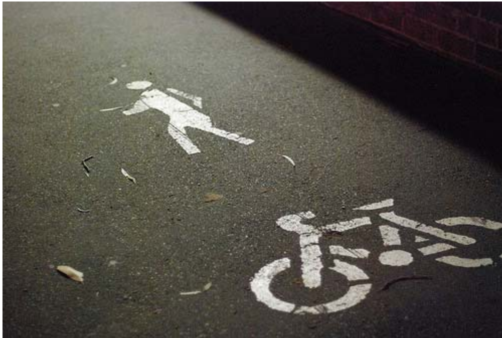
Figure 5 - Example of shared path pavement markings
