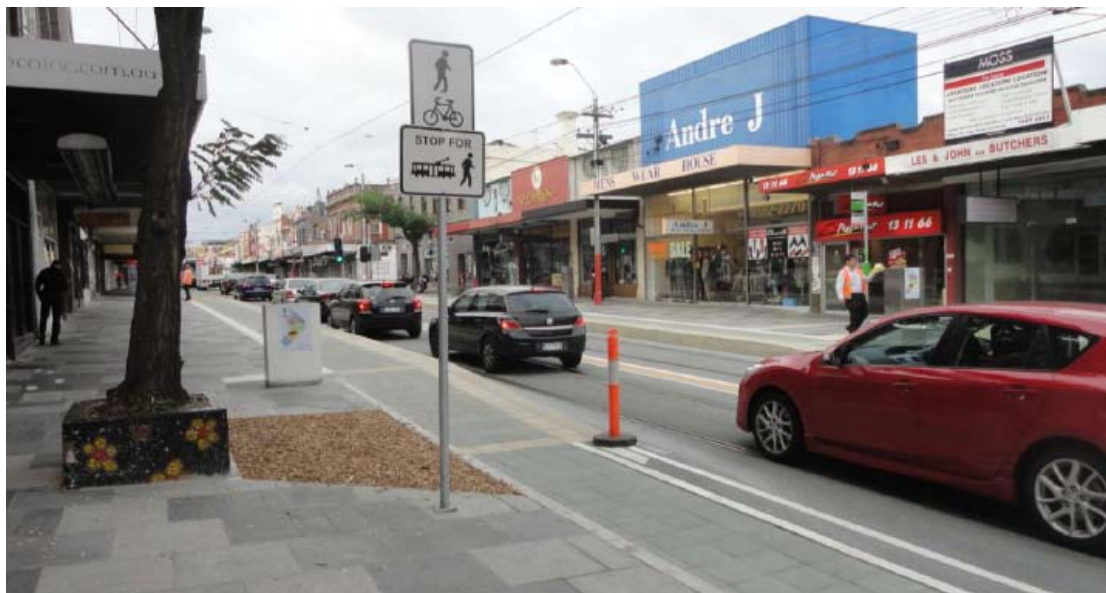
Figure 3 - Shared path at tram stop 32
