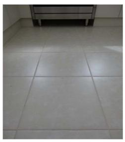
Ceramic tiles with epoxy grout
