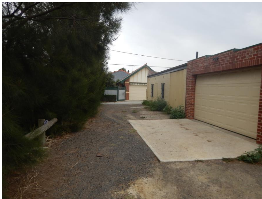
41 and 43 Cameron Street, as viewed from the laneway to the north of the site, April 2016
