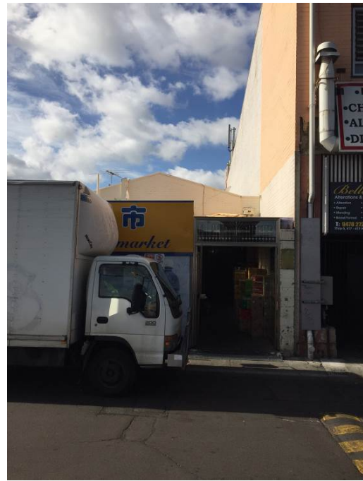
Figure B.3 – 2016 Photo – 421 High Street (rear)
