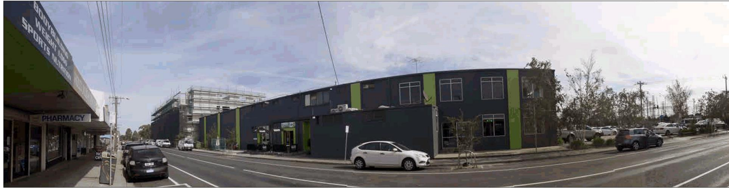
STREETScape JOHNSON STREET - FACING SUBJECT SITE
