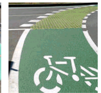
No Buffer painted cycle lane- Gold Coast (Streetbond)
