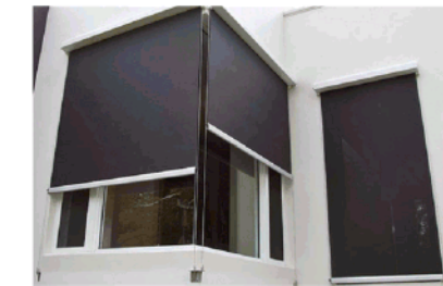
EXTERNAL ROLLER BLIND (ERB) DETAILS ERB EXTERNAL ADJUSTABLE ROLLER BLINDS (MANUAL CRANK OPERATION) TO ALL NORTH, EAST AND WEST FACING HABITABLE ROOM WINDOWS/GLAZED DOORS
