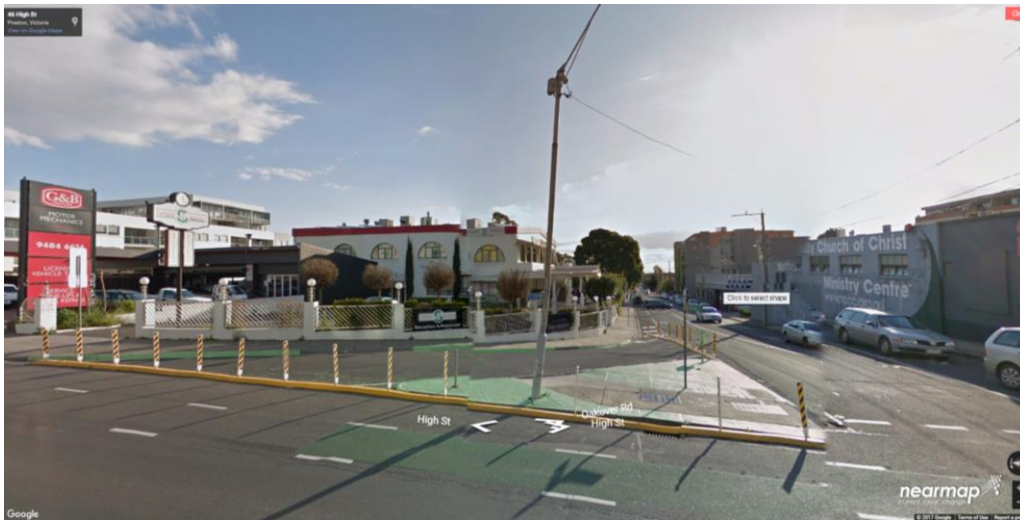
Figure 1: Temporary closure of the Oakover Road slip lane.
