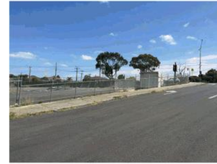
SHARED ACCESS ROAD LOOKING TO PLENTY ROAD VICROADS SUBSTATION
