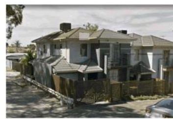
ACCESS ROAD FROM SLIP LANE
