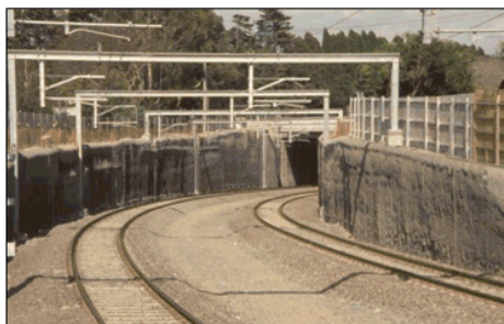
Figure 4: A lowered rail line at Middleborough Rd, Box Hill
