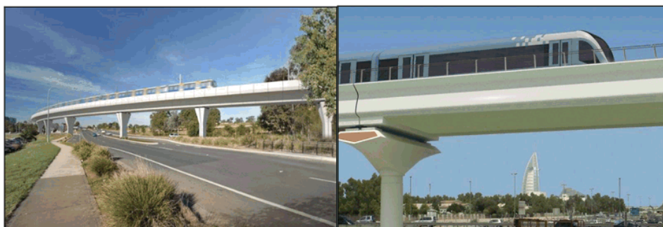
Figure 3: Examples of elevated rail lines – Sydney metro North West ( left ) and Dubai Metro ( right )
