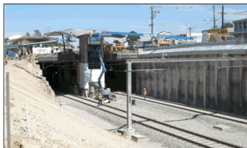
Figure 5: Construction during the rail line lowering at Springvale Rd, Springvale
