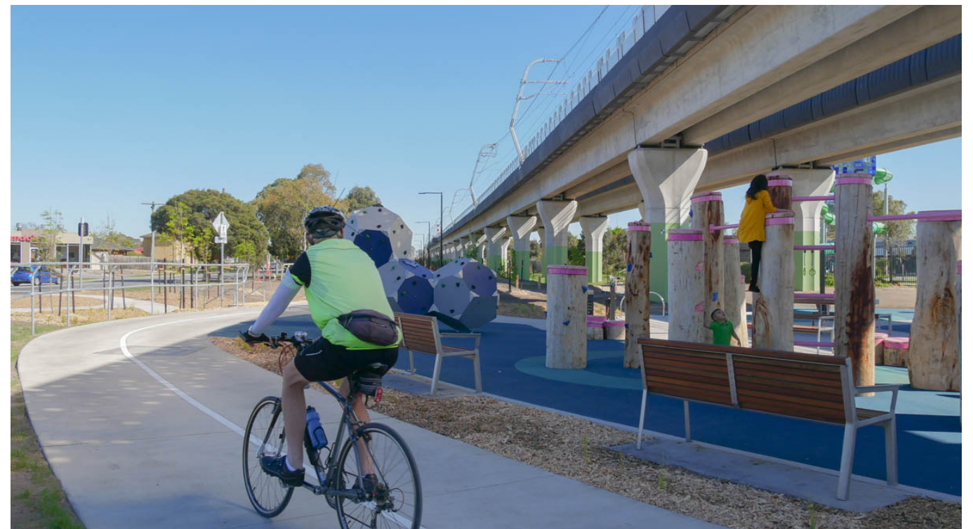
Shared User Path connecting into surrounding active transport links. Source: LXRP
