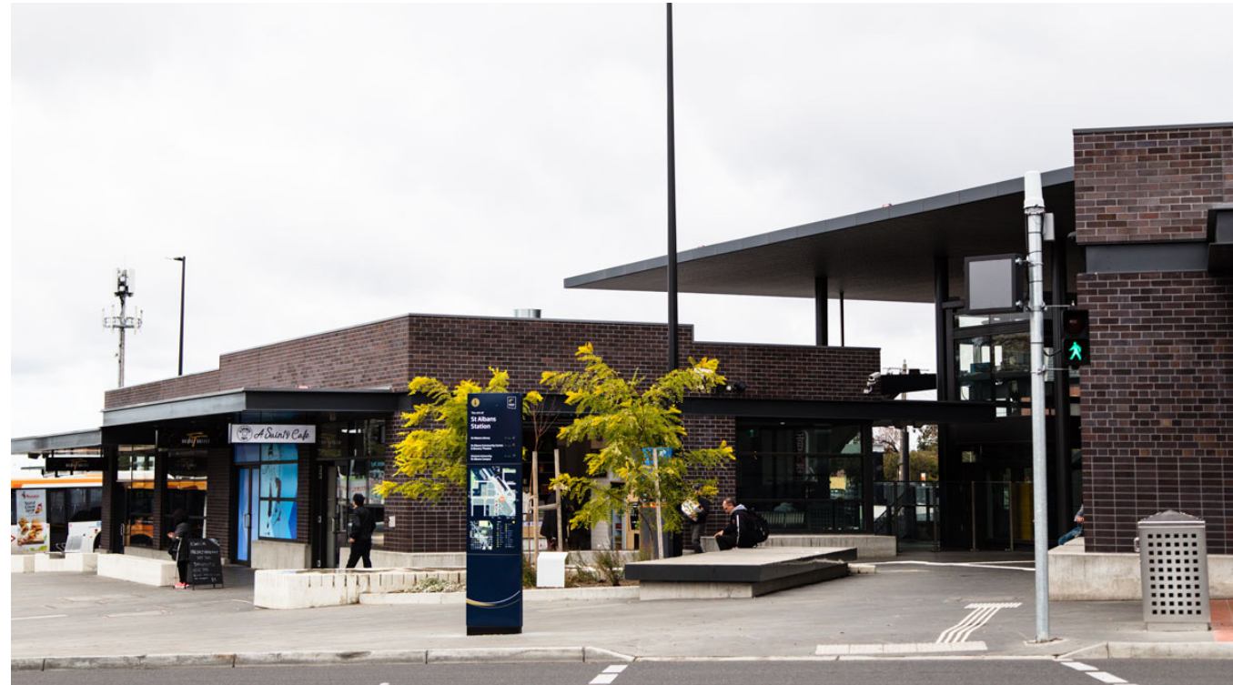
St Albans Station entry activated with retail frontages. Source: LXRP
