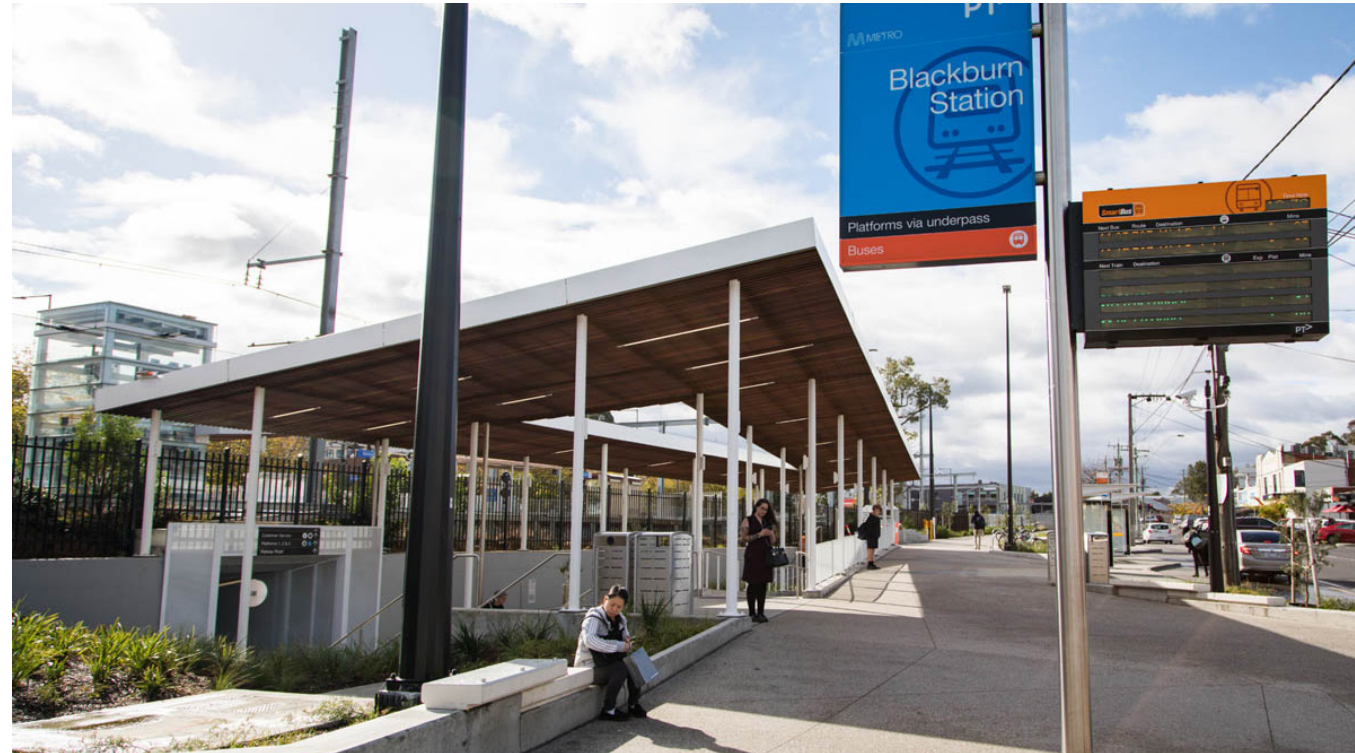
Integrated bus interchange at Blackburn Station. Source: LXRP
