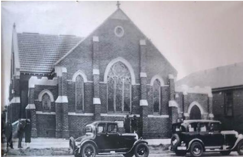
Figure 3. C. 1930s view of the Croxton Methodist Church, looking north. Note the vents on the roof of the Sunday School. Source: Social media post (Facebook, Croxton Uniting Church).
