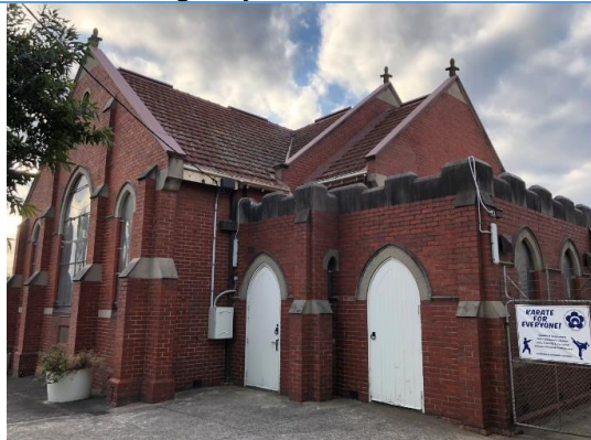
Oblique overview of the southern elevation and rear of the church. Source: Extent Heritage Pty Ltd, 2024.
