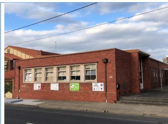
Oblique view of the Community Hall façade, looking northeast. Source: Extent Heritage Pty Ltd, 2024.
