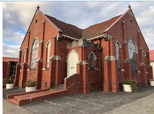
Entrance to the Methodist Church, looking northeast, showing the western and southern gables. Source: Extent Heritage Pty Ltd, 2024.
