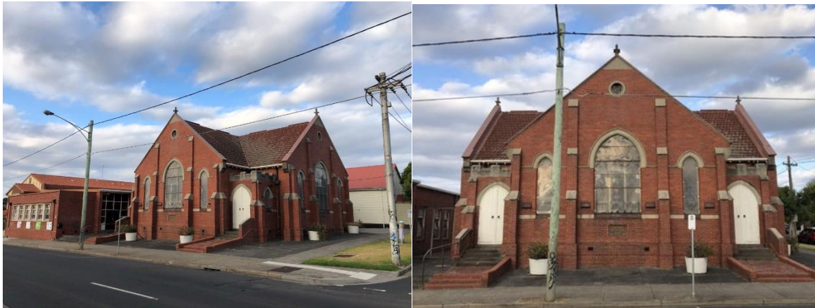
Figure 1 Former Croxton Methodist Church
