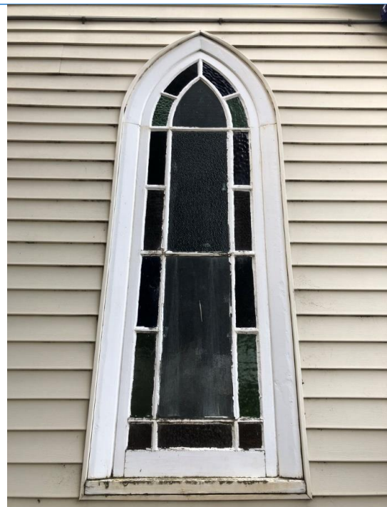
Eastern lancet window on the Church Hall façade. Source: Extent Heritage Pty Ltd, 2024.
