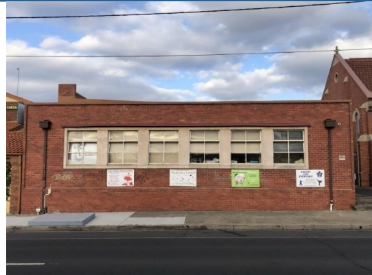
Direct view of the Community Hall façade, looking east. Source: Extent Heritage Pty Ltd, 2024.
