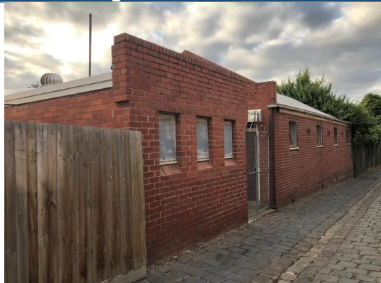
Oblique overview of the Kindergarten and 1958 toilet block, looking northwest. Source: Extent Heritage Pty Ltd, 2024.
