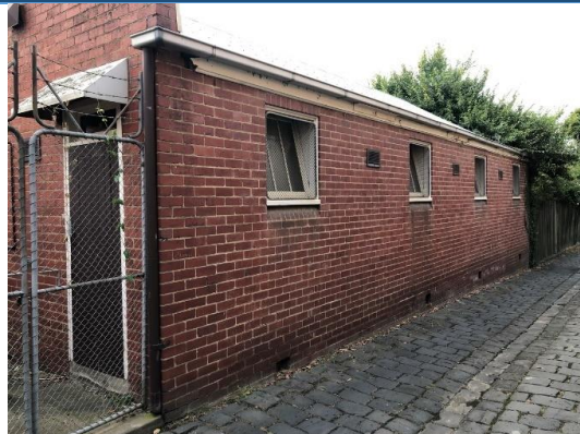
Oblique overview of the Kindergarten looking northwest. Source: Extent Heritage Pty Ltd, 2024.
