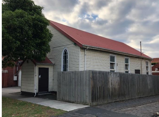
Northwestern view of the 1912 Former Church Hall. Source: Extent Heritage Pty Ltd, 2024.
