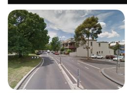
A T-intersection with kerb outstands is intended to reduce speeds of throughtraffic. The treatment comprises kerb outstands on the through-road.
