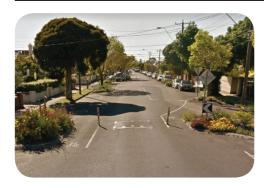
A pinch point is intended to reduce vehicle speeds. The treatment comprises kerb extensions to narrow the trafficable width to 3.5 m (one lane) and may also include a centrally located road cushion to slow vehicular traffic.
