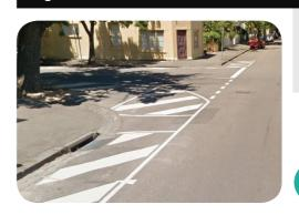
A semi-mountable area with contrasting material is intended to provide a visual effect to reduce speeds of vehicles approaching an intersection.
