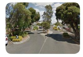
A chicane is intended to reduce vehicle speeds. The treatment comprises kerb extensions to narrow the trafficable width to 3.5 m (one lane) and provides an angled traffic lane to slow vehicular traffic. This treatment also includes bicycle sharrows to warn motorists of cyclists and to encourage cyclists to take the lane.
