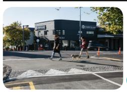
A raised side street treatment (with optional kerb outstands) is intended to reduce vehicle speeds on approach to intersections with collector roads. The treatment comprises a flat top road hump on the discontinuing leg of a T-intersection to slow vehicular traffic, as well as optional kerb outstands on the main road to separate on-street car parking. This treatment can be used with or without on-street bicycle lanes.
