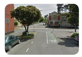
Contra-flow bicycle lanes are exclusive bicycle lanes deployed on one side (to the left of the opposing traffic flow) of a one-way road serving cyclists travelling against what is otherwise the legal direction of travel. Physical separation between the contra-flow bicycle lane and the traffic lane should be considered where vehicle speeds are 60 km/h or greater.
