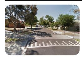
A raised shared path crossing is intended to reduce vehicle speeds to the pedestrian / cyclist crossing point and raise the awareness of the potential conflict point. The raised profile will require motorists to reduce speeds through the crossing. It is desirable to provide kerb extensions to create a pinch point to further slow vehicle speeds and to reduce the crossing point.
