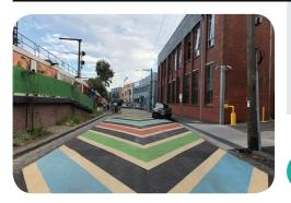
A shared zone is intended to reduce vehicle speeds and provide equal priority to pedestrians, cyclists and vehicles. The treatment generally comprises a contrasting road pavement and a 10 km/h speed limit.
