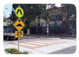
A raised wombat crossing is intended to allocate priority to crossing pedestrians and reduce vehicle speeds. The treatment comprises kerb extensions to narrow the trafficable width to 5.5 m and a zebra crossing to allocate pedestrian priority on top of a flat top road hump to slow vehicular traffic
