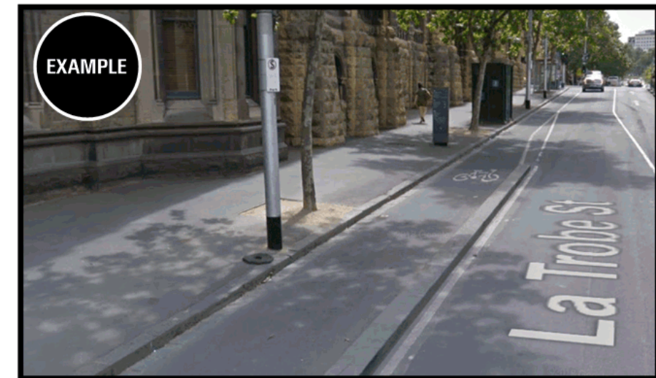
Example of protected cycle lane with raised kerb to improve cycling confidence along La Trobe Street, Melbourne.
