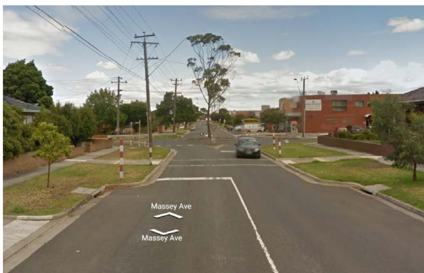
Figure 2 Existing Massey Avenue School crossing
