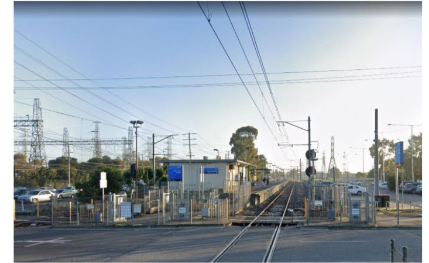
Poor rail interface. Source: Google Maps Street View
