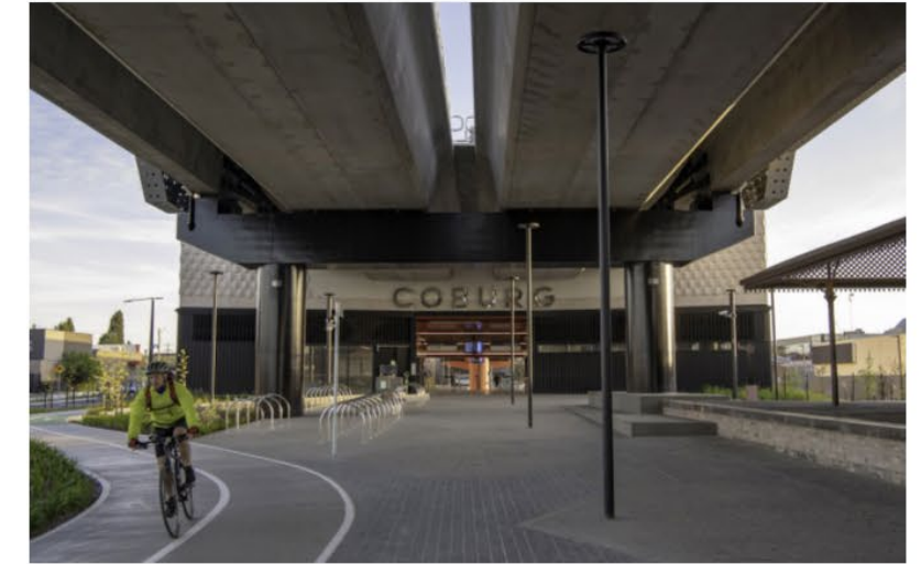
Active transport links underneath the rail bridge. Source: LXP
