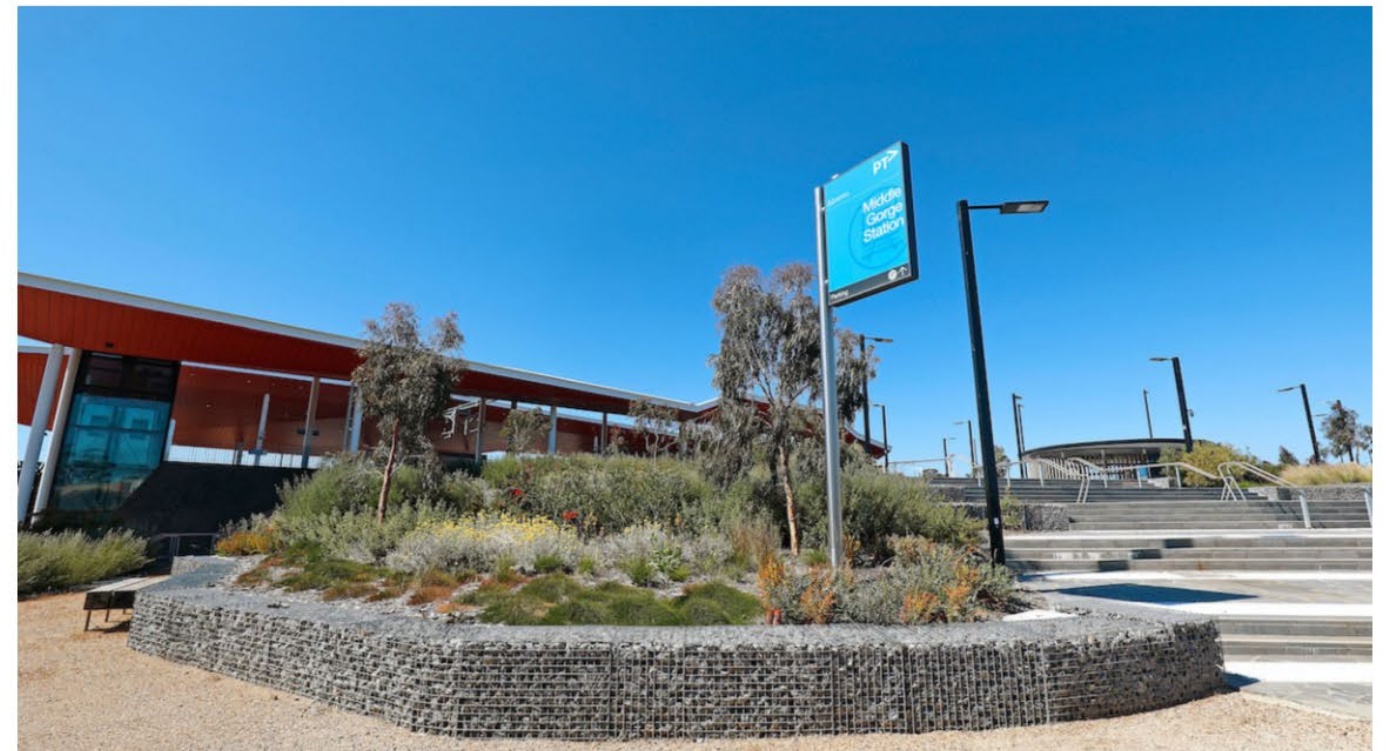
Complementary materials at Middle Gorge Station. Source: LXRP
