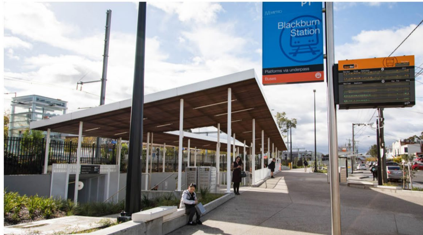
Integrated bus interchange at Blackburn Station. Source: LXP
