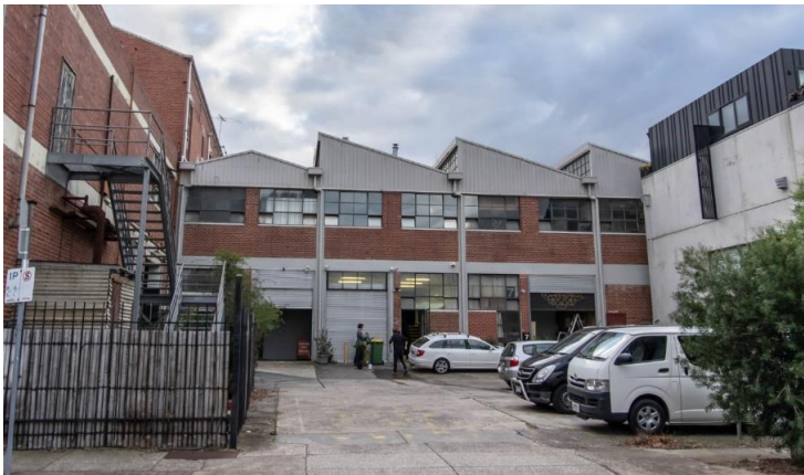
Figure 20. East elevation of Building 7 viewed from Westgarth Street. Note the original metal-frame windows and saw tooth roofs highly legible on this elevation. (Source: Context, May 2020)
