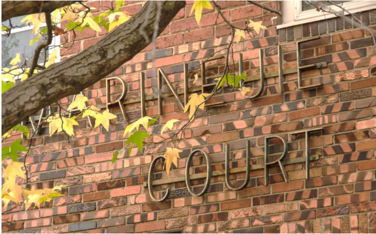
Figure 4. Showing the thin metal signage 'Marineuie Court' and brickwork incorporating clinker brick and varigated tapestry brick. (Source: Context, May 2020)
