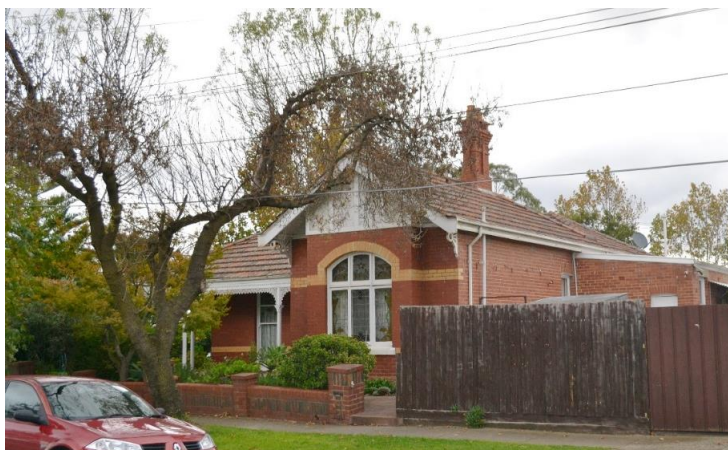
Figure 1. 607 Heidelberg Road, Alphington. (Source: Context, May 2020)
