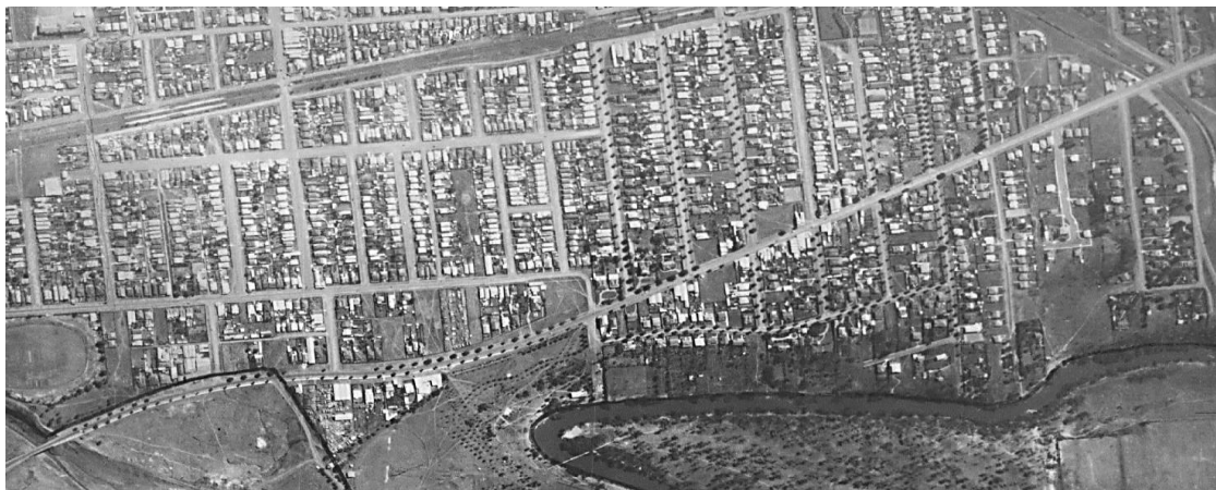
Figure 4. A section of a 1931 aerial photograph showing Heidelberg Road between Merri Creek and Grange Road. The development of industrial sites was observed around the western end of the study area, while the middle section (around today’s Fairfield) was developed with residences and small-scale commercial or industrial sites. (Source: Central Plan Office, ‘MALDON PRISON (11/1931)’, via Landata)
