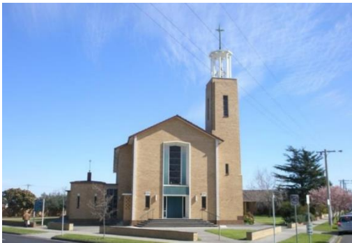
Figure 17. St Gabriel's Catholic Church Complex at 237-243 Spring Street, Reservoir (HO280).
