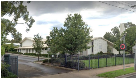
Figure 12. LDS Church in Glenroy Road, Glenroy (No HO). (Source: Google, February 2020)
