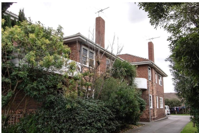
Figure 1. East elevation of 441 Heidelberg Road, Fairfield. (Source: Context, May 2020)
