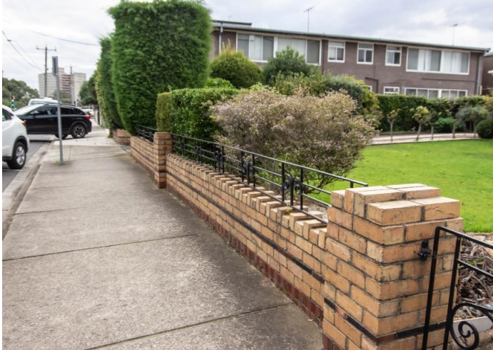
Figure 6. Details of the front fence of 257 Heidelberg Road, constructed of matching cream brick laid in header course with brown and dark red brick accents. Mild steel gates and fence panels are also original. (Source: Context, May 2020)
