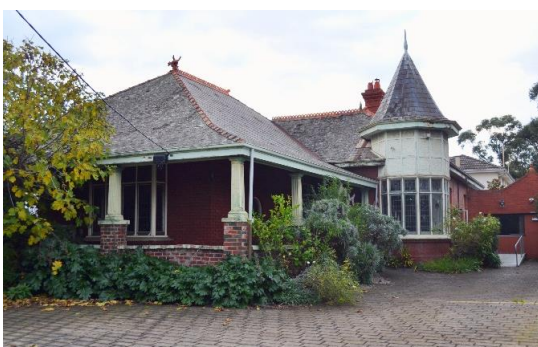
Figure 7. 331-333 Heidelberg Road, Northcote (recommended for inclusion in the Darebin Planning Scheme Heritage Overlay in the Heidelberg Road Heritage Assessment, Context 2020)
