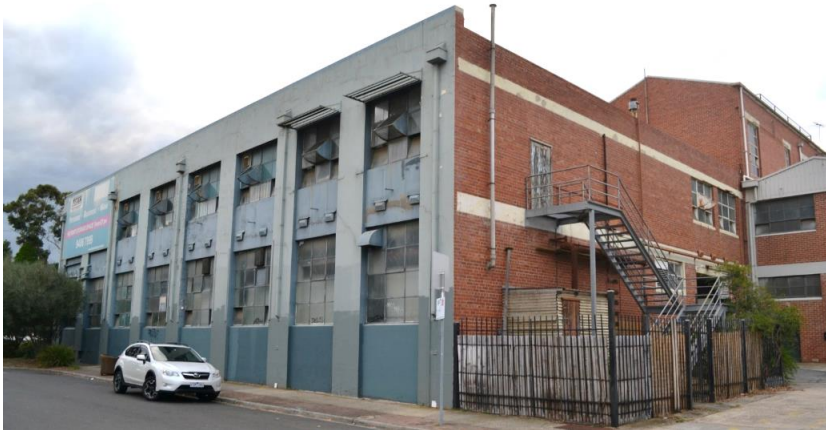
Figure 14. Westgarth Street and rear (north) elevation of Building 1. The Westgarth Street elevation features intact large multi-pane windows divided by narrow pilasters. The north elevation is of face brickwork with less glazing and intact upper level windows and doors. (Source: Context, May 2020)
