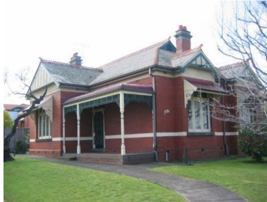
Figure 4. 'Balleer' 648 Bell Street, Preston (HO204).
