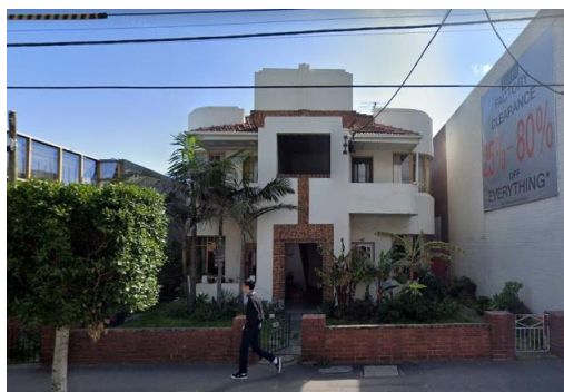
Figure 14. 301 Lygon Street, Brunswick East (Serial Listing HO443, City of Moreland). (Source: Google, September 2019)
