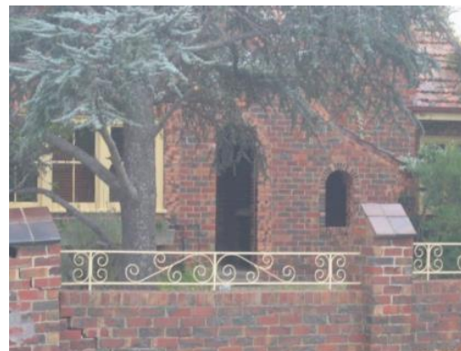
Figure 19. Close up of 18 Barton Street, Reservoir, showing the portico entrance.
