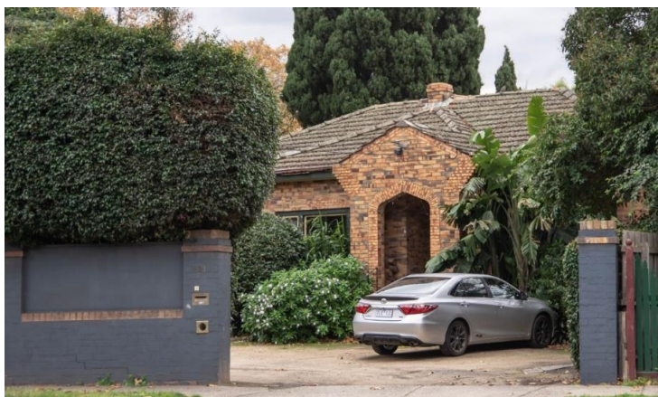
Figure 16. Southern elevation of 521 Heidelberg Road, Alphington.
