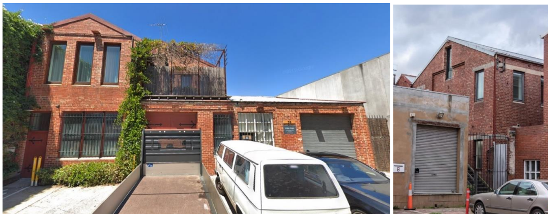
Figure 18. C.1909-31 Building 6 on the northwest corner of the site (left-hand side) and its rear elevation (right-hand side). (Source: Google, February 2020; Context, May 2020)
