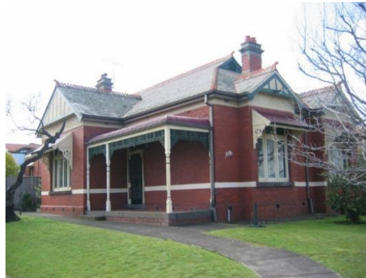
Figure 4. 'Balleer' 648 Bell Street Preston (HO204).
