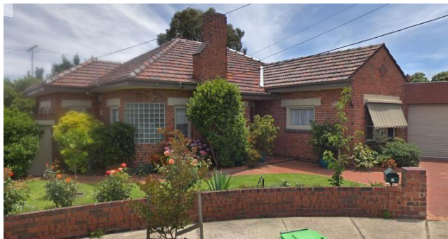
Figure 10. 9 Kelley Grove, Preston, in the Kelley Grove Precinct (HO103). (Source: Google, December 2018)
