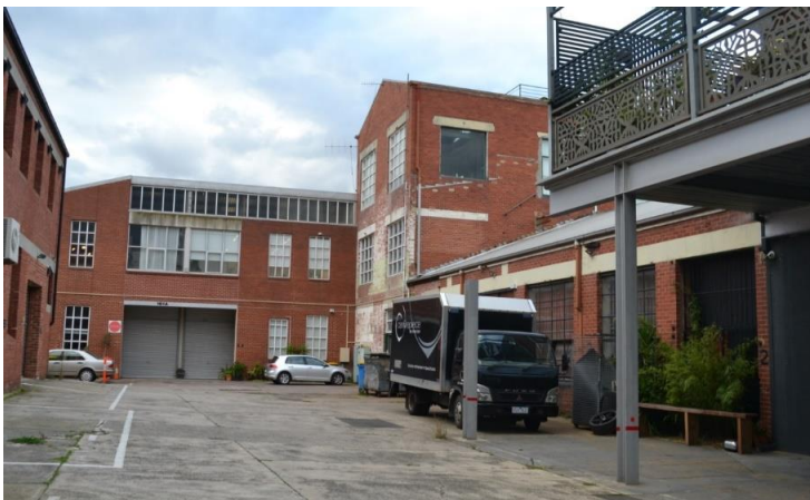
Figure 21. View into the site from Heidelberg Road, showing the new south wall of Building 7, rebuilt after 1981 following partial demolition (left-hand side); Building 7's three-storey gabled wing with new glazing (middle); earlier single-storey Building 2 behind Building 1 (right-hand side); and the steel-frame balcony added to Building 1 (far right). (Source: Context, May 2020)
