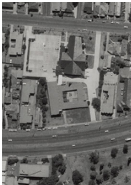
Figure 8. 273-289 Heidelberg Road in January 1981. Note the passage between the earlier building and the new chapel was completed by this time. (Source: Central Plan Office, 'WESTERN PORT FORESHORES (1/1981)' via Landata)
