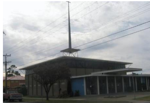
Figure 16. St George's Anglican Church, 32-34 Ralph Street, Reservoir (HO279).
