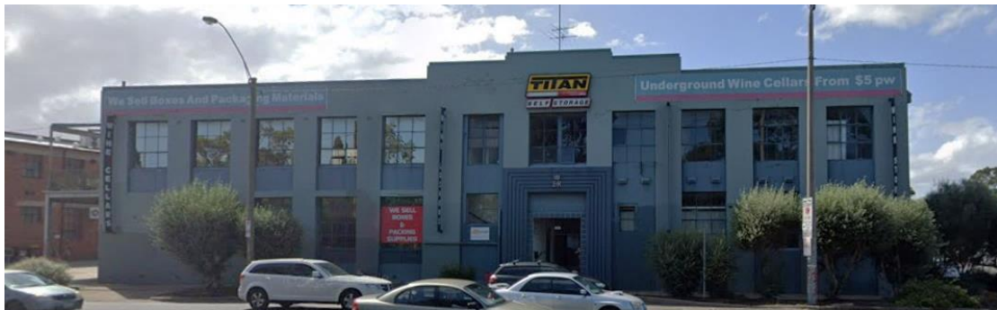
Figure 12. The main building (Building 1) at the corner of Heidelberg Road and Westfield Street, built in 1939. (Source: Google, February 2020)
