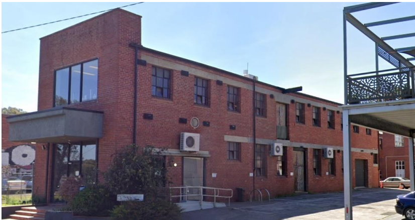
Figure 15. C.1939 Building 3 at the southwest corner of the site. The east elevation appears largely original. (Source: Google, February 2020)
