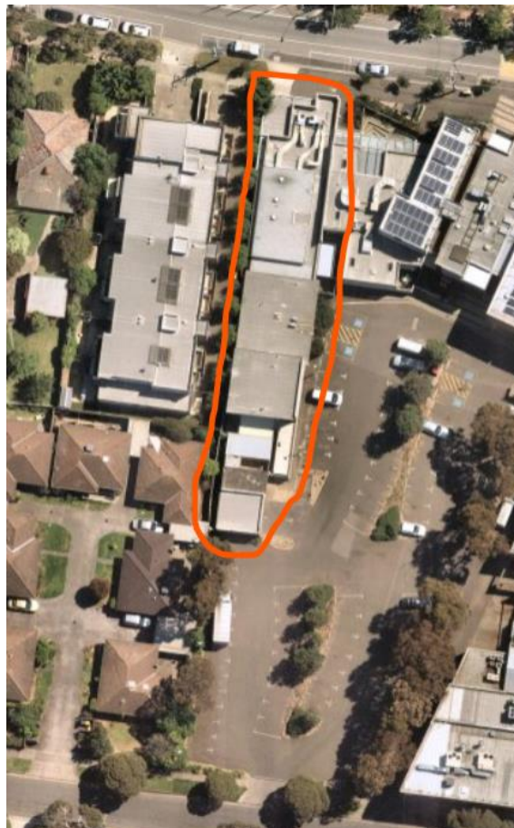
Figure 1 Aerial view of 25 Edwardes Street Reservoir - Nearmap
