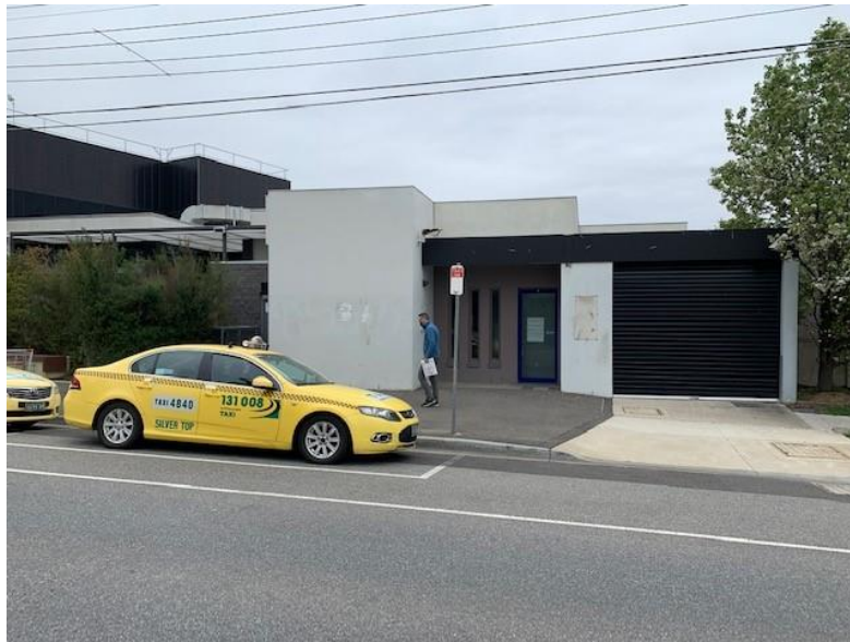
Figure 2 Street view of 25 Edwardes Street Reservoir
