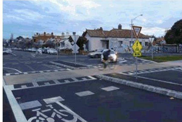
High quality raised crossings, designed to accommodate people and bikes. Source: VicRoads
