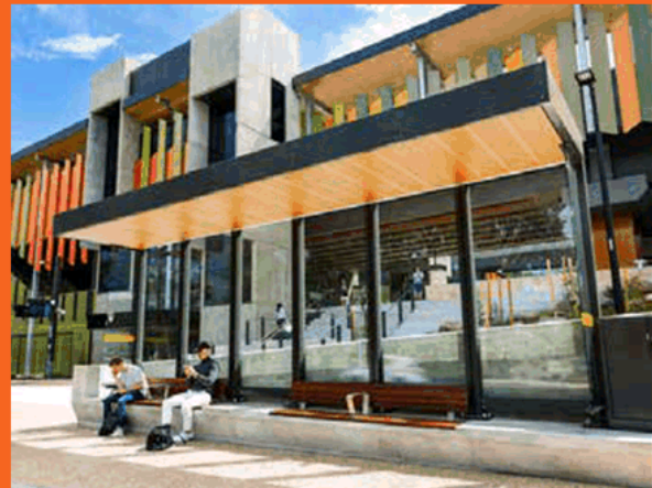
Custom bus shelters should be easily accessible from the new entry to Preston and Bell Stations
