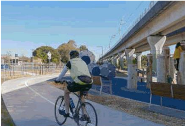
Meandering shared user path to support local trips underneath the new elevated rail corridor. Source: Level Crossings Removals Project website
