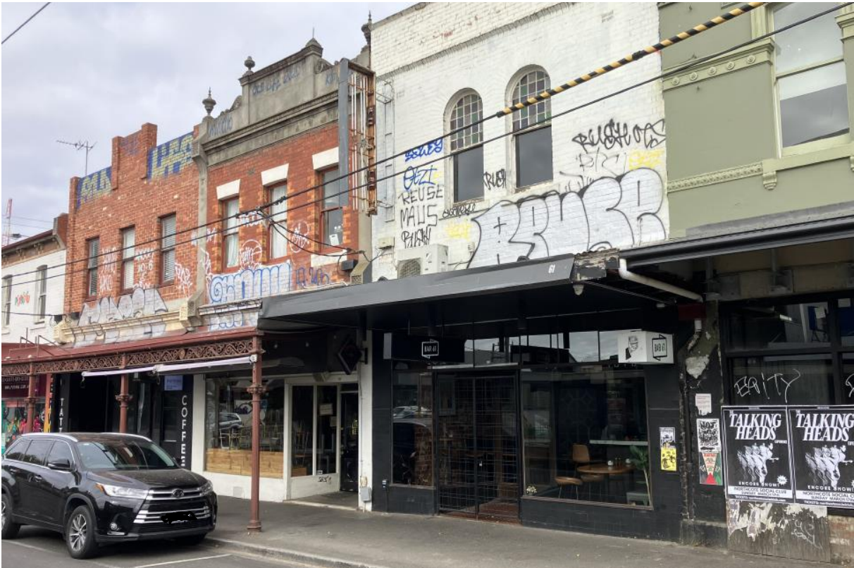
Figure 1: Subject site viewed from east Source: Author
