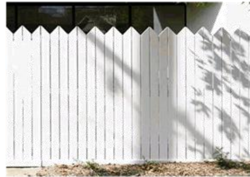
P2 -70x19 mm WHITE PAINTED TIMBER PICKET FENCE WITH 20MM SPACING LOCATION -SOUTH CRES / WASTELL STREET FRONT FENCES FRONT FENCE TYPE 1
