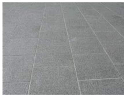
P12 -CONCRETE PAVERS CHARCOAL GREY LOCATION -UPPER LEVEL BALCONIES
