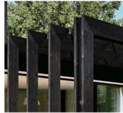
P3 -BLACK PAINTED TIMBER LOCATION - GARAGE ARBOUR STRUCTURES
