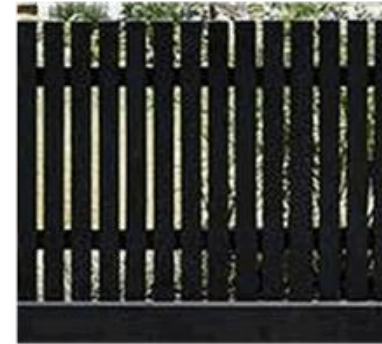
P14 -70x19 mm BLACK PAINTED TIMBER PICKET FENCE WITH 20MM SPACING LOCATION -FRONT FENCE TYPE 2
