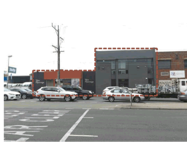
02 SUBJECT SITE - 345-349 BELL ST.
