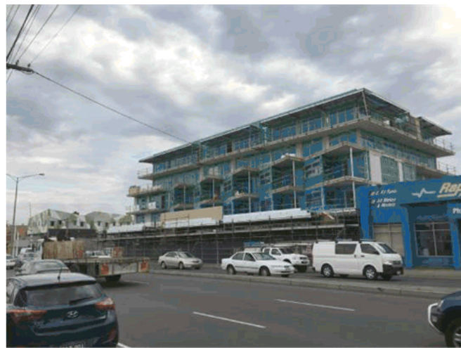
04 352 BELL ST. 6 LEVEL MIXED USE DEVELOPMENT UNDER CONSTRUCTION
