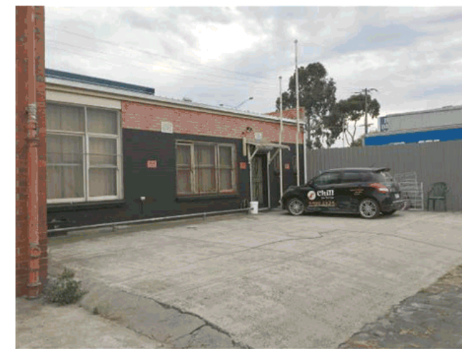
11 SUBJECT SITE - 345 BELL ST. VIEW FROM R.O.W.
