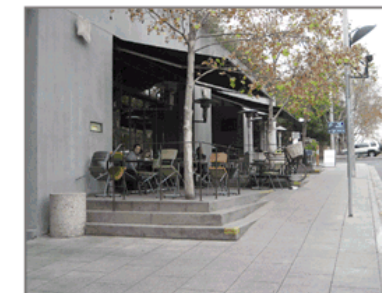
Benchmark Image F Level changes are well handled, simple and consistent ground plane treatment and provision of shade with trees and canopies create attraction and comfortable pedestrian amenity
