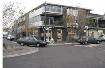
Benchmark Image D Corner buildings should have greater height to define the corner. Buildings should be articulated and provide active edges
