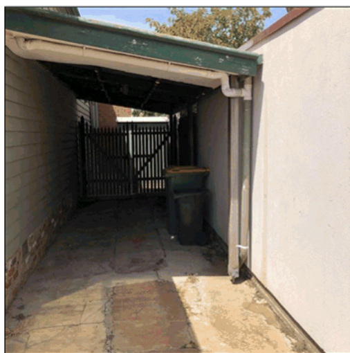
Figure 3 – existing garage structure
