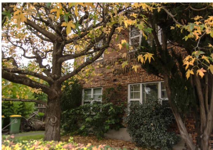
Figure 2. South elevation of 441 Heidelberg Road, Fairfield. (Source: Context, May 2020)
