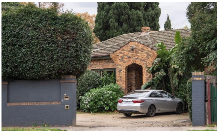
Figure 16. Southern elevation of 521 Heidelberg Road, Alphington.
