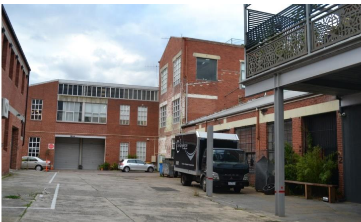
Figure 21. View into the site from Heidelberg Road, showing the new south wall of Building 7, rebuilt after 1981 following partial demolition (left-hand side); Building 7's three-storey gabled wing with new glazing (middle); earlier single-storey Building 2 behind Building 1 (right-hand side); and the steel-frame balcony added to Building 1 (far right). (Source: Context, May 2020)
