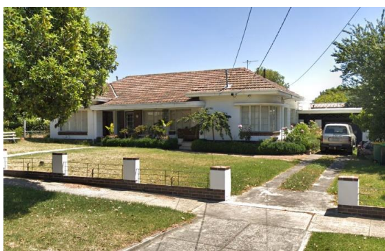
Figure 7. 36 Cooper Street, Preston (HO208). (Source: Google, July 2019)
