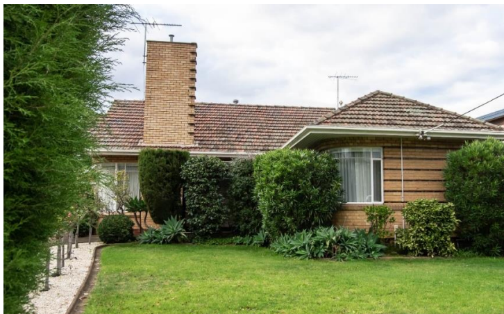
Figure 1. 257 Heidelberg Road, Northcote. (Source: Context, May 2020)
