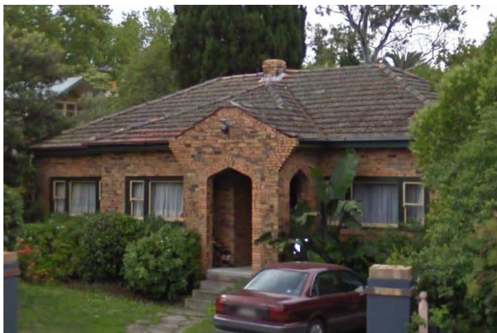
Figure 17. Southern elevation of 521 Heidelberg Road, Alphington in 2009 showing fenestration and second portico opening. (Source: Google, 2009)
