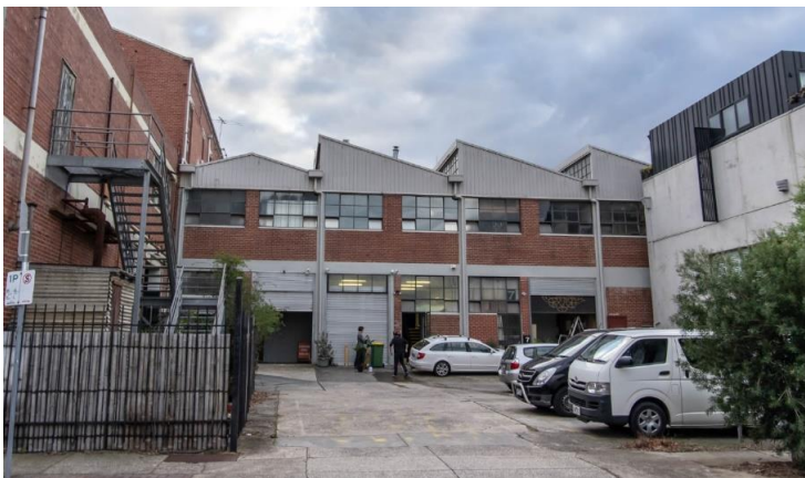
Figure 20. East elevation of Building 7 viewed from Westgarth Street. Note the original metal-frame windows and saw tooth roofs highly legible on this elevation. (Source: Context, May 2020)
