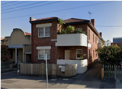
Figure 11. 423 Canning Street, Carlton North (significant in HO326 North Carlton Precinct, City of Yarra). (Source: Google, November 2019)
