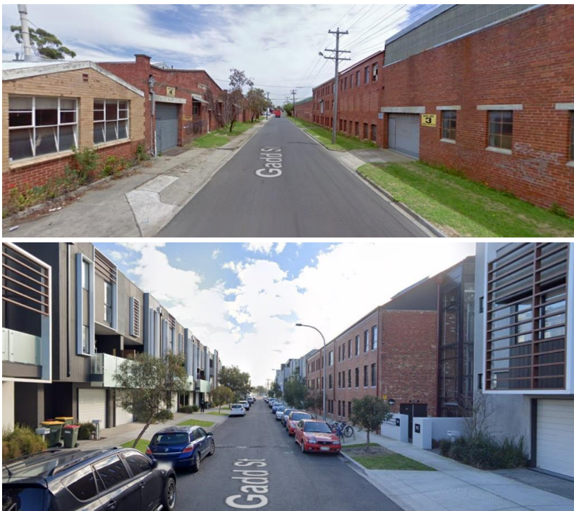
Figure 25. Former Joshua Pitt Pty Ltd Tannery (HO180) at 52-60 and 71 Gadd Street, Northcote in 2009 (upper) and 2019 (lower). Buildings on both sides have been demolished, and the surviving building from the early twentieth century was converted to apartments. (Source: Google, November 2009; July 2019)
