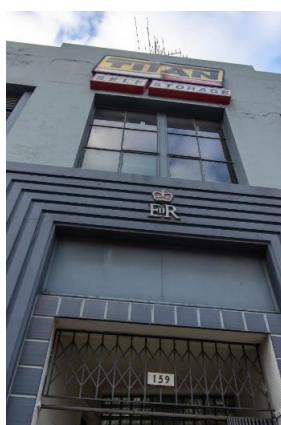
Figure 13. The Royal cypher above the entrance of the Building 1. Note the distinctive oversized stepped architrave around the front entrance that is inset with tiled edges. (Source: Context, May 2020)
