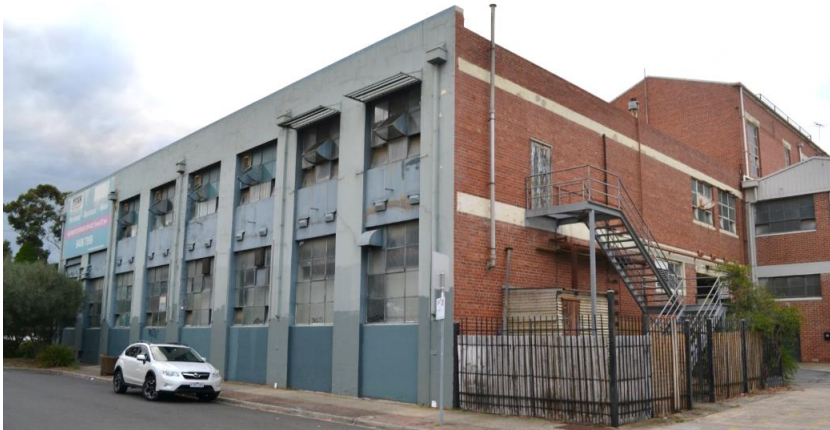
Figure 14. Westgarth Street and rear (north) elevation of Building 1. The Westgarth Street elevation features intact large multi-pane windows divided by narrow pilasters. The north elevation is of face brickwork with less glazing and intact upper level windows and doors. (Source: Context, May 2020)
