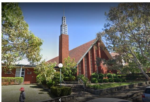
Figure 14. LDS Church in Greenwich Road, Greenwich, New South Wales. (Source: Google, November 2019)
