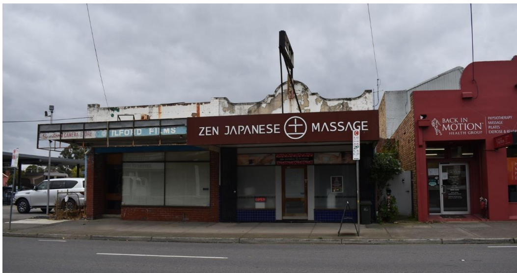
Figure 17: View of 727 (left) and 729 (right) Heidelberg Road (source: Extent Heritage)
