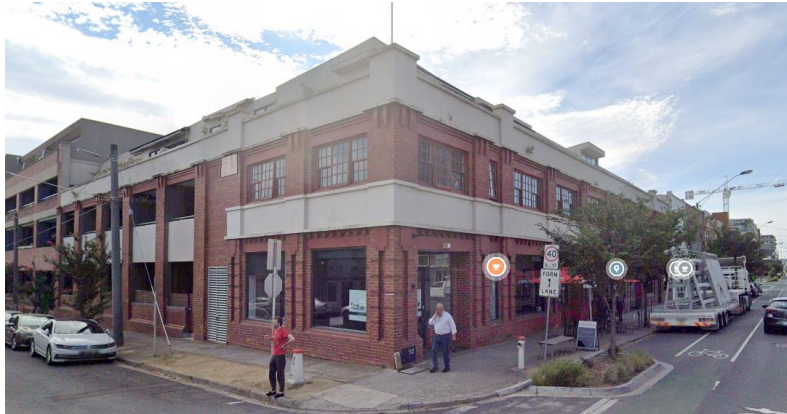
Figure 35: View of the former Howe Leather Factory (source: Google Streetview)
