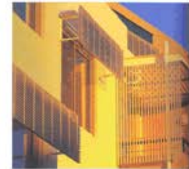
Benchmark Image I Pergolas and screens to provide sun protection and privacy
