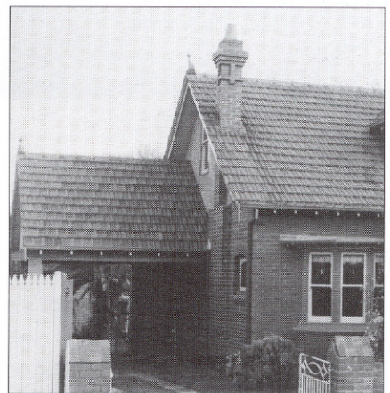
Car port attached to the side of a Federation bungalow using roof form and design elements of the original house.
