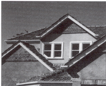
Roof form is critical. Matching roof materials, pitch, gable details, as well as a matching chimney have produced a convincing attic alteration and addition.
