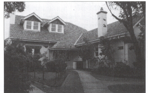
Addition and alterations have reproduced original English style elements and used matching materials and finishes.
