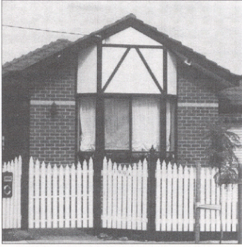
Contemporary interpretation of traditional design elements – scale, setback, roof form and pitch, bay window, gable with half timbered effect and traditional materials. Inclusion of brick chimney makes the result more convincing.
