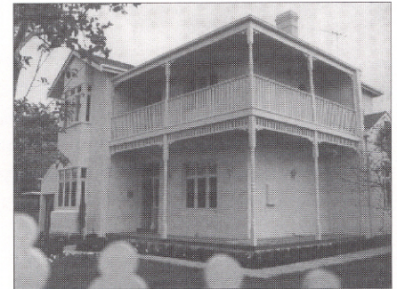
Interpretation of Federation House. Traditional red brick with roughcast render has been replaced by rendered brick.
