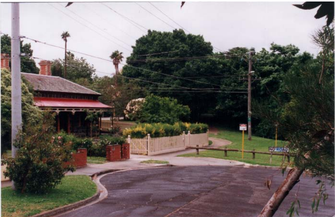
2.6 “Mayville”, erected by John May c.1872, overlooks the treeclad Merri Creek valley at the east end of Cunningham Street.
