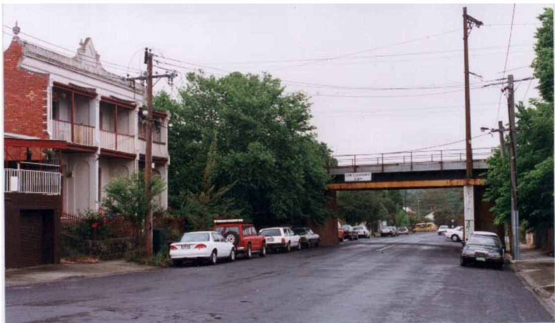
2.4 Urquhart Street, looking east to the railway viaduct.
