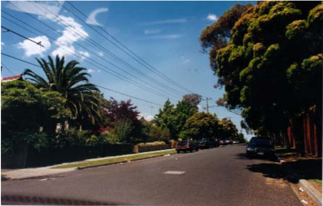
Hawthorn Road. The wall of the former Little Sisters of the Poor is at right.
