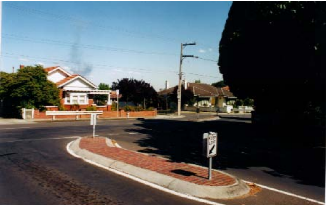
The King William Street/Oakhill Avenue intersection showing the traffic management devices that impact negatively on the Garden Suburb character of the Area.
