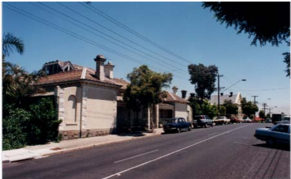
The Mitchell Street slope with the Salvation Army citadel in the distance.
