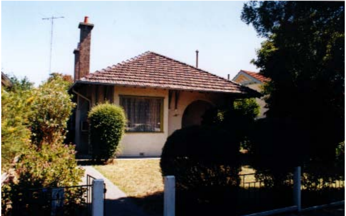
No.11 Adeline Street is a substantially intact example of the distinctive Arts and Crafts cottage imparting significance to the Area.
