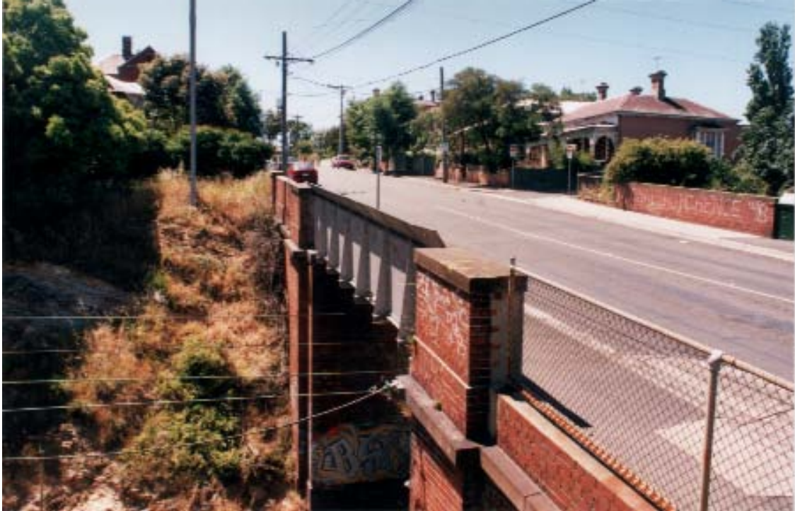
The Westbourne Grove road bridge over the railway.
