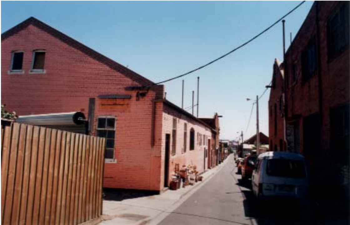
Eastment Street, looking north.
