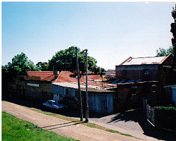
40 Shaftsbury Prade - showing former dairy
