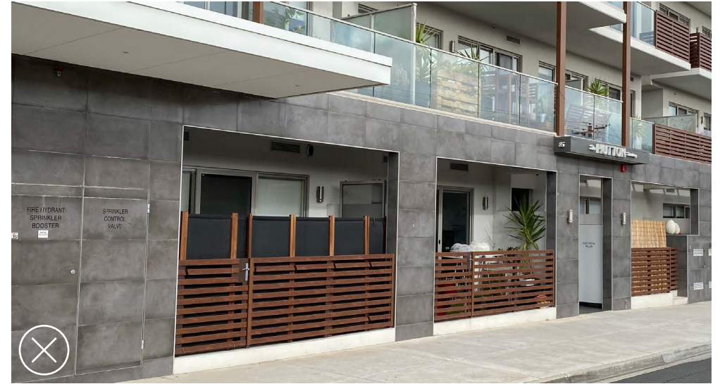
Ground floor residential interface with zero setback results in high screening or close blinds compromising internal amenity and passive surveillance.
