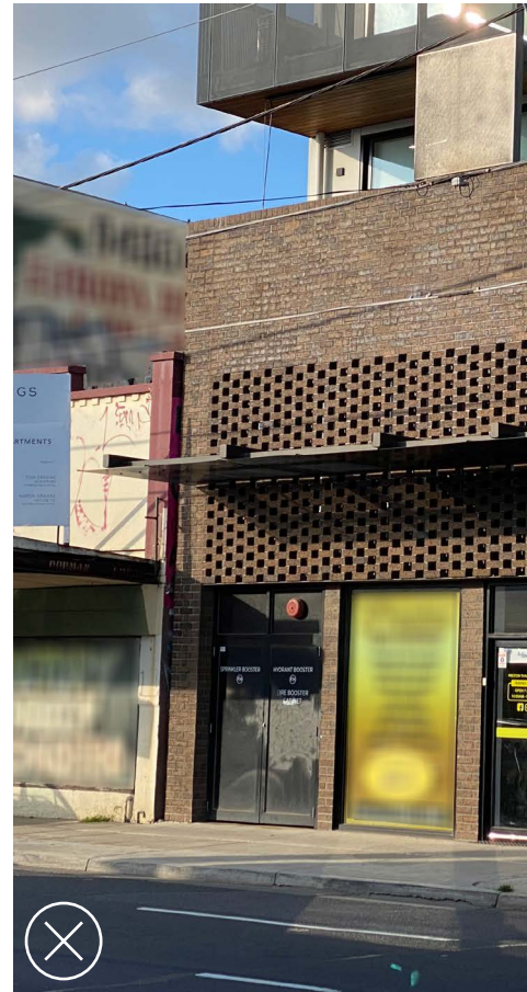
Awnings that are high are inconsistent in the streetscape and do not provide adequate weather protection.
