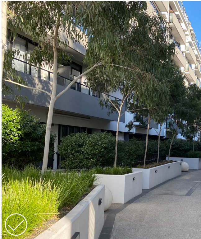
Planter beds for trees should include appropriate soil based on the species and size of the tree to ensure they will grow to optimum size.
