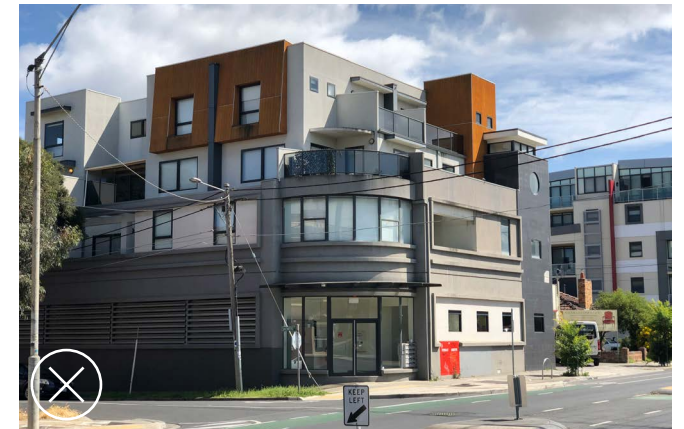
Too many materials with different colours create a cluttered and confused facade.
