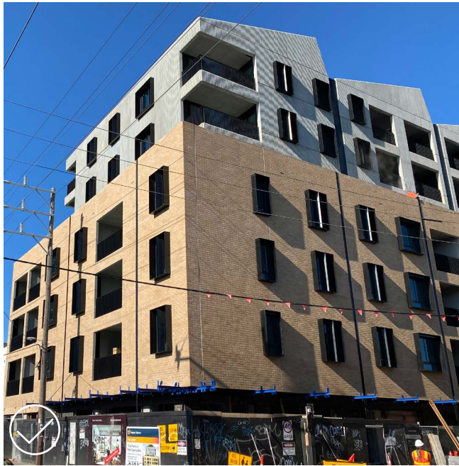
Large upper level setback along with change in material clearly defines the street wall.
