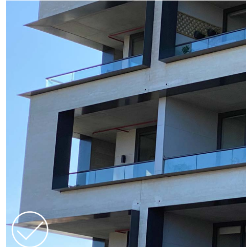
Part concrete with glass on top
