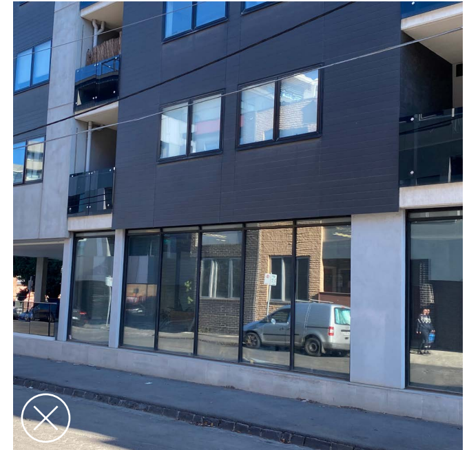
Large expanse of reflective glass without any articulation does not provide interaction between the building and the street.
