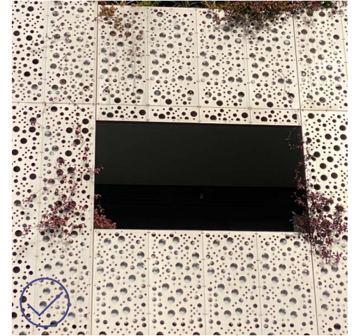
Laser cut steel cladding
