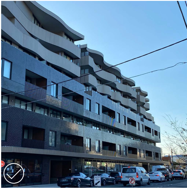
Contrasting building articulation along with change in material and upper level setback creates a visually dominant street wall
