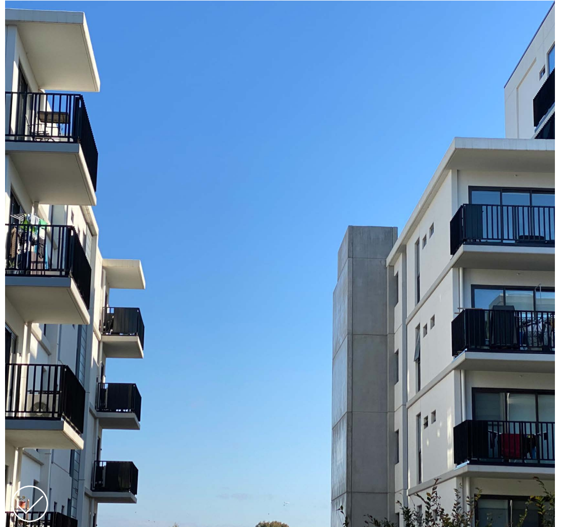
Orienting balconies in different direction can help redirect the view and achieve privacy without the need for high privacy screens.
