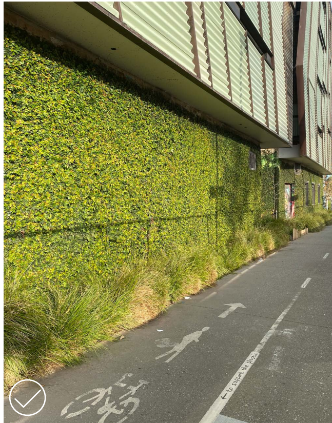
✓ Creepers along the wall can provide greenery and also reduce graffiti on the wall.
