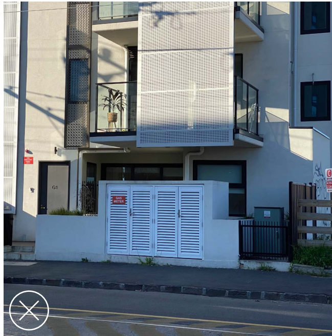
Free standing services enclosed in a box can be a barrier and compromise ground level amenity
