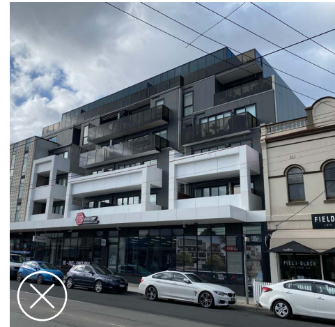
Insufficient upper level setback and poor material selection can result in inconsistent street wall.
