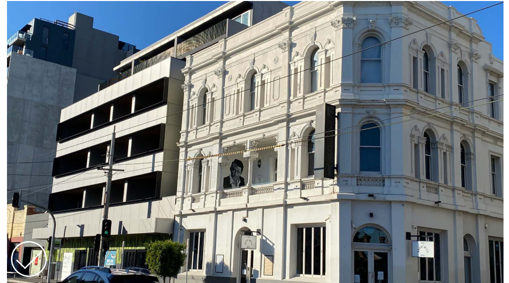
Consistent street wall creates a pedestrian friendly scale and character.
