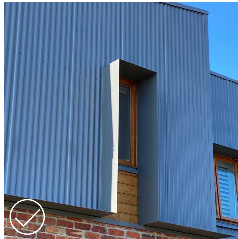
Small and protected windows or windows with louvered screens can help reduce solar gain on the western facade.
