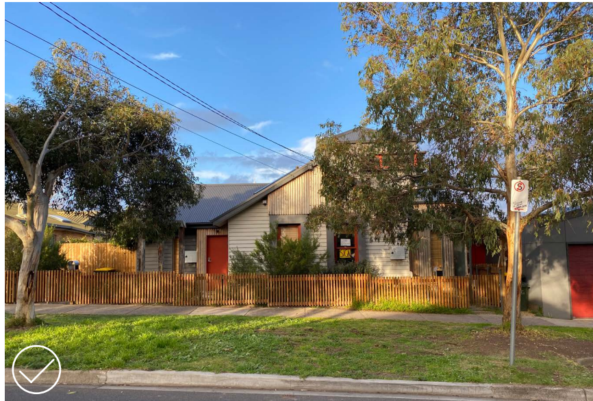
Development with integrated roof form and landscaping creates a side by side development that presents as one dwelling with two separate entrances.
