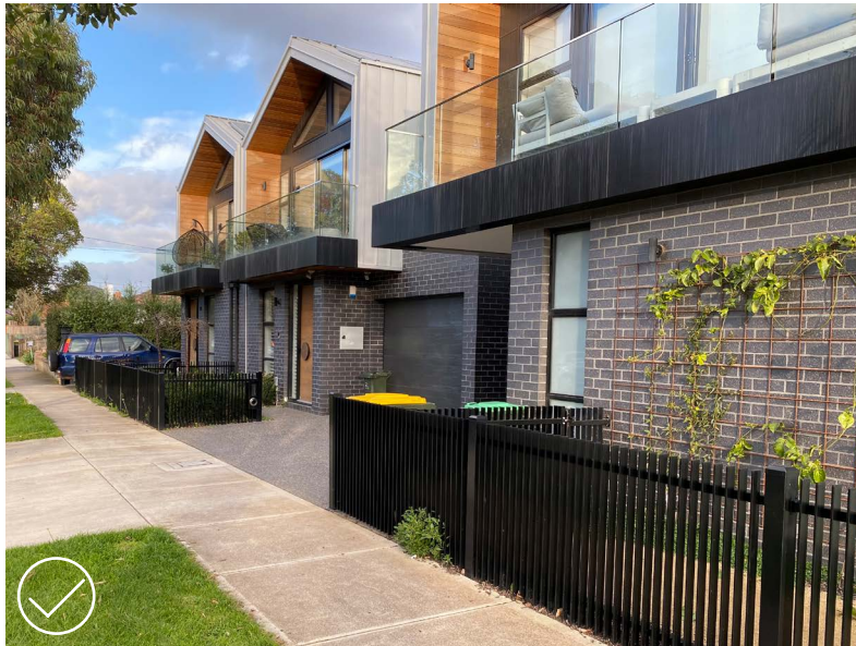
Recessed garages reduce their dominance and highlight the buildings and clearly visible dwelling entry.
