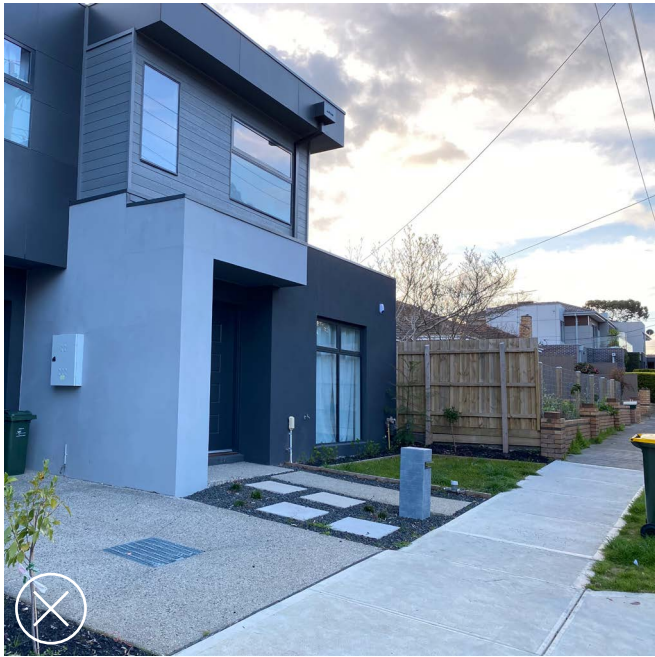
Poor landscaping and transition between the dwelling and the footpath impacts amenity of the dwelling.
