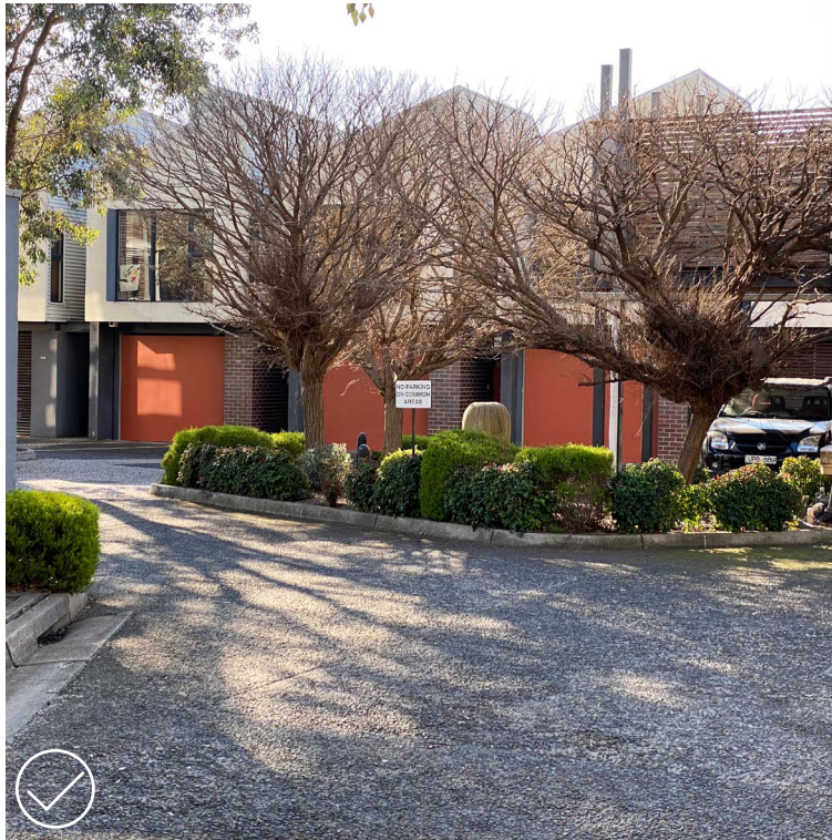
Driveways designed as shared space with textured materials and landscaping can create a pedestrian friendly environment.
