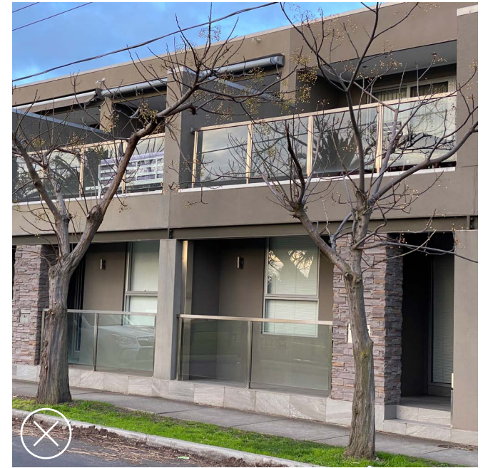
Lack of appropriate ground level setback results in poor amenity for residents with blinds drawn down majority of the time.
