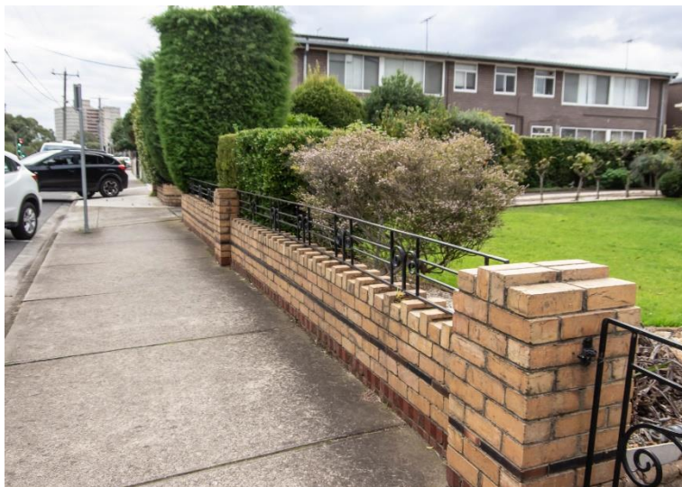
Figure 6. Details of the front fence of 257 Heidelberg Road, constructed of matching cream brick laid in header course with brown and dark red brick accents. Mild steel gates and fence panels are also original. (Source: Context, May 2020)
