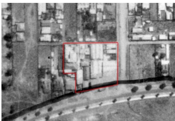
Figure 4. Subject site in 1931, fully developed with buildings. (Source: Central Plan Office, 'MALDON PRISON (11/1931)', via Landata)
