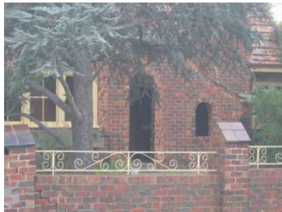
Figure 19. Close up of 18 Barton Street, Reservoir, showing the portico entrance.
