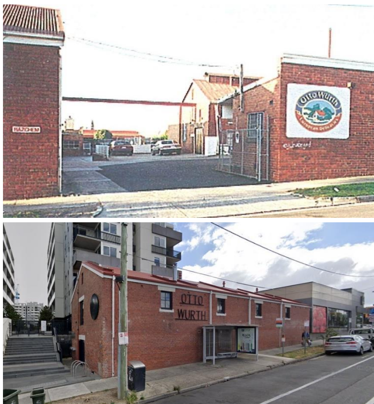
Figure 22. Former Watson & Paterson Bacon-Curing Factory (HO30), at the corner of Dundas Street and Plenty Road, Preston c.2000 (upper) and in 2019 (lower).
