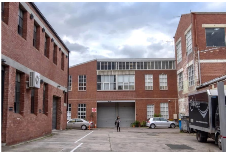
Figure 2. View into the site from Heidelberg Road. (Source: Context, May 2020)
