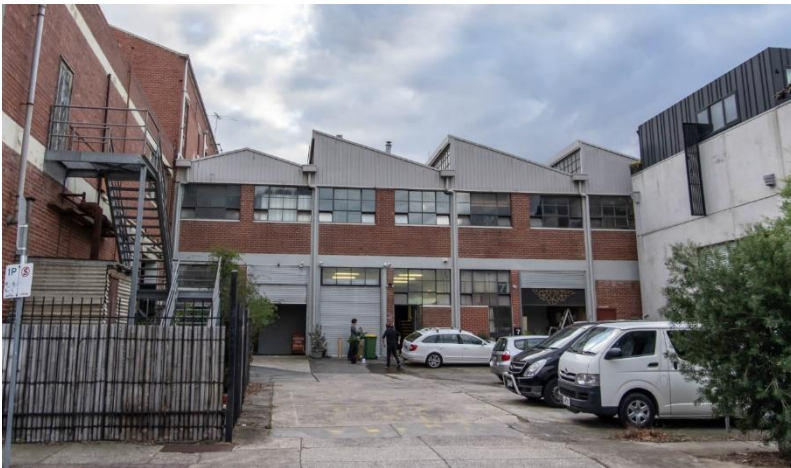
Figure 20. East elevation of Building 7 viewed from Westgarth Street. Note the original metal-frame windows and saw tooth roofs highly legible on this elevation. (Source: Context, May 2020)
