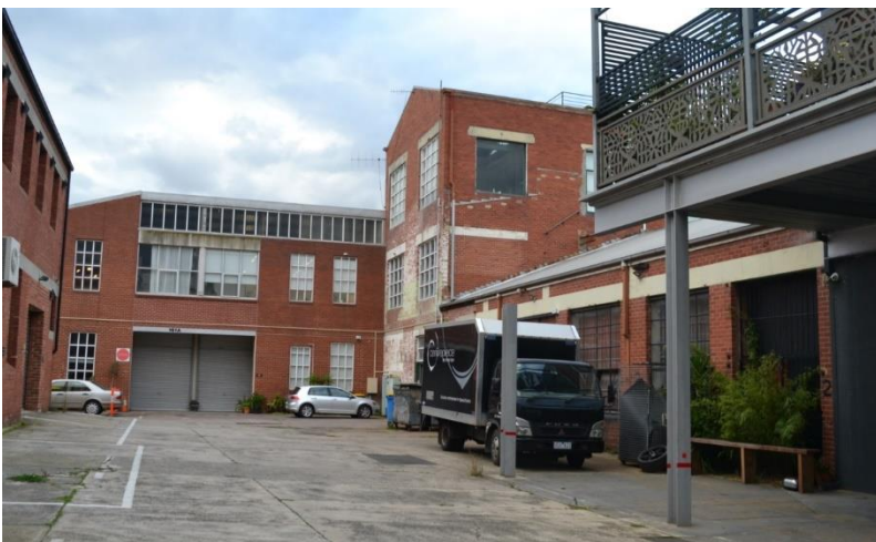
Figure 21. View into the site from Heidelberg Road, showing the new south wall of Building 7, rebuilt after 1981 following partial demolition (left-hand side); Building 7's three-storey gabled wing with new glazing (middle); earlier single-storey Building 1 behind Building 1 (right-hand side); and the steel-frame balcony added to Building 1 (far right). (Source: Context, May 2020)
