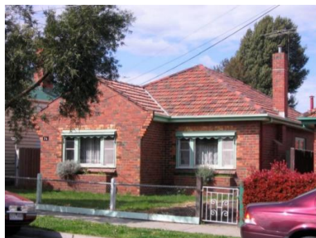
Figure 24. 26 William Street, Preston, C1 graded in the 'Heart of Preston' (William Street) Precinct (HO183).
