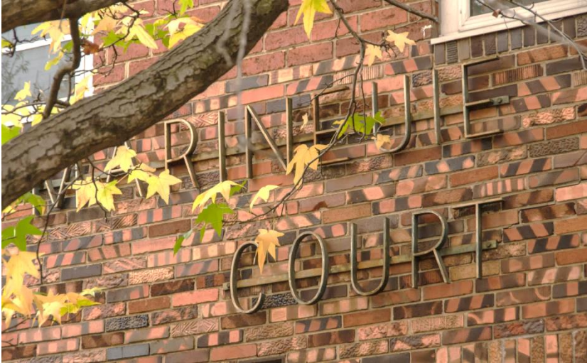
Figure 4. Showing the thin metal signage 'Marineuie Court' and brickwork incorporating clinker brick and varigated tapestry brick. (Source: Context, May 2020)
