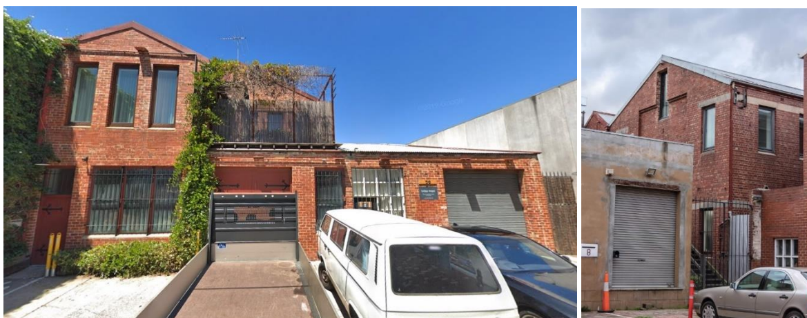
Figure 18. C.1909-31 Building 6 on the northwest corner of the site (left-hand side) and its rear elevation (right-hand side). (Source: Google, February 2020; Context, May 2020)
