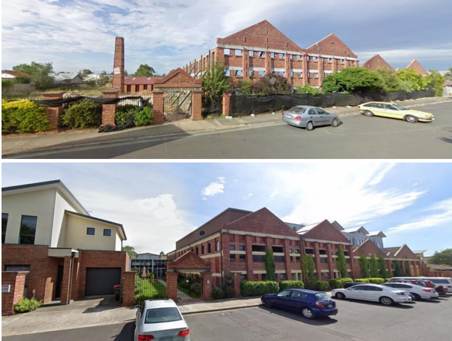
Figure 24. Former Northcote Pottery (HO176) at 85a Clyde Street, Thornbury during the demolition work in late 2009 (upper) and after conversion into apartments in 2019 (lower). (Source: Google, December 2009; January 2019)
