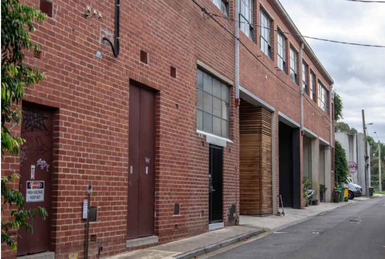
Figure 19. View along Albert Street, Showing the c.1939 Building 7 with some intact ground-level detailing (left-hand side) and new ground-level openings (right-hand side). (Source: Context, May 2020)
