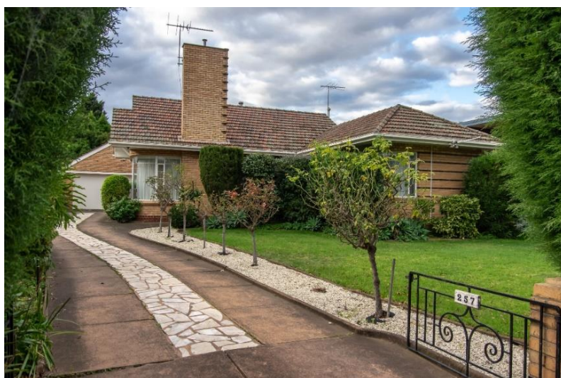
Figure 2. 257 Heidelberg Road, Northcote, looking into the front gate. (Source: Context, May 2020)
