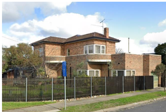
Figure 8. 499 St Georges Road, Thornbury (assessed and recommended as individually significant place in 'Thornbury Park Estate Precinct' 2020). (Source: Google, July 2019)
