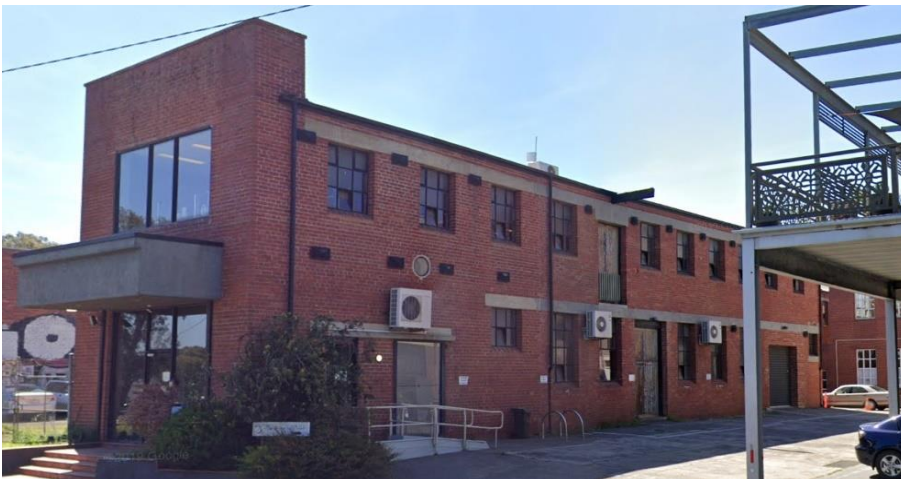
Figure 15. C.1939 Building 3 at the southwest corner of the site. The east elevation appears largely original. (Source: Google, February 2020)
