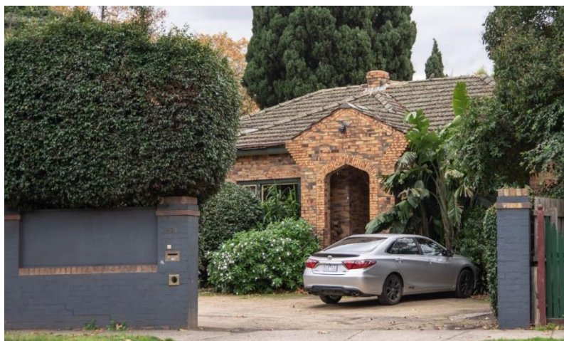
Figure 16. Southern elevation of 521 Heidelberg Road, Alphington.
