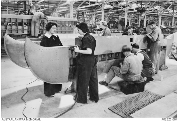
Figure 3. Women assembling a Beaufort tail plane at the Department of Aircraft Production's Beaufort Division complex, c.1942. (Source: Australian War Memorial, via Darebin Heritage)
