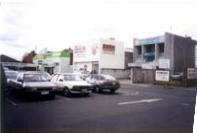
Existing unsafe & unattractive car parks
