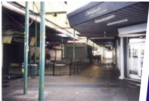
Existing unsafe & illegible pedestrian link to station
