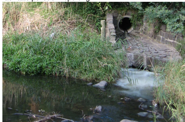
A polluted stormwater drain north of Blyth Street, Brunswick East
