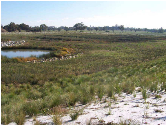
Photo 3 - Campbellfield Creek Retarding Basin wetland development
