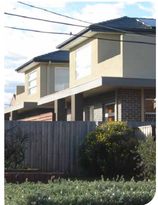
Existing medium density development in the Reservoir MAA
