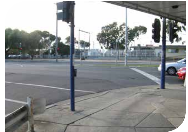
Opportunities to provide signalised pedestrian crossings on both sides of Edwardes Street and Broadway to provide better access into the station precinct
