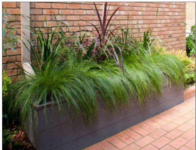
Figure 9 - Raingarden planter boxes can be installed above ground where opportunities for ground-level planters are limited
