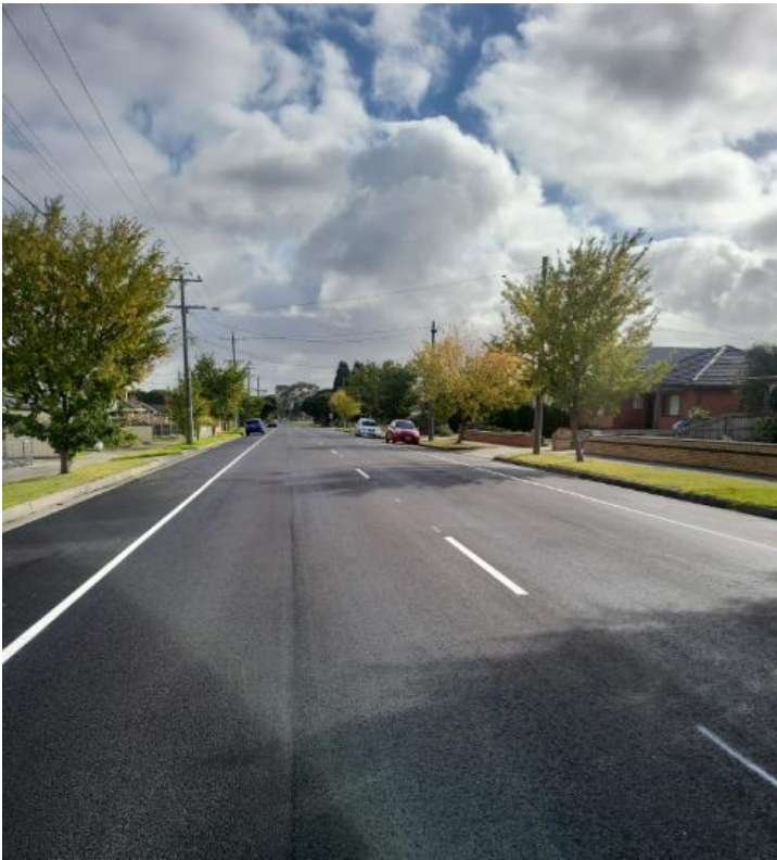
Pictured: New road surface at Allenby Avenue, Reservoir.
